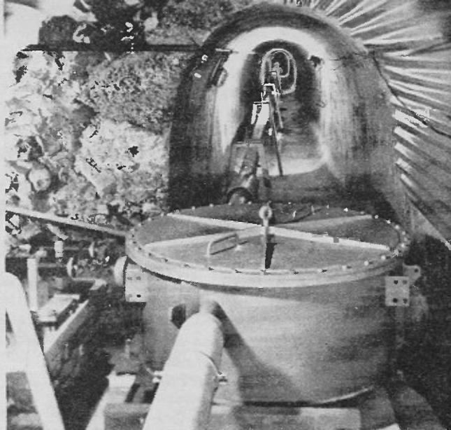
Fig. 11. The University of Trieste laser earth strain meter.
