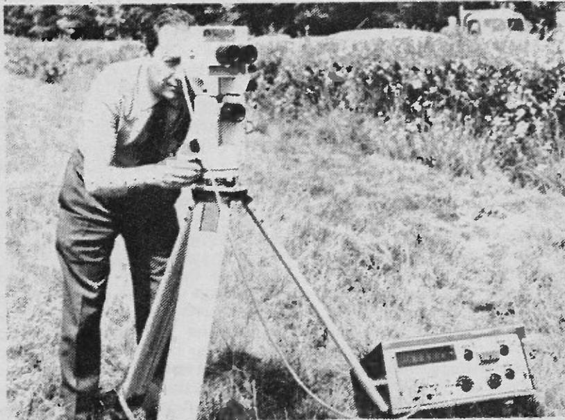
Fig. 14. Gallium-arsenide diode powered transit time ranger.
