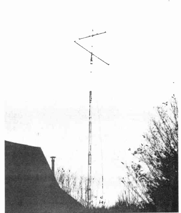
G4LJF's 100ft tower with KT34XA and KLM yagi for 40m
