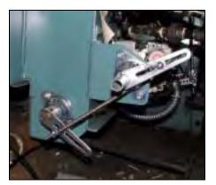
Figure 4-4 Rotary air damper linkage at low fire position
