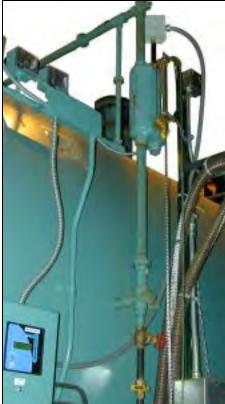
Figure 2-1. Water Column with Level Master
