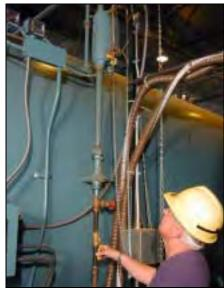
Figure 2-10. Blowing Down the Water Column
