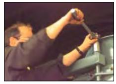
Figure 2-12 Tighten Davit Nut
