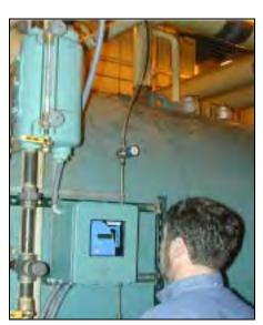
Figure 1-10 Water Column and Level Master Low Water Cut-Off
