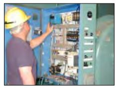
Figure 5-3 Flame Safety Inside Burner Control Panel
