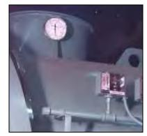
Figure 2-7 Stack Thermometer
