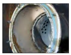
Figure 1-5 Access Way to Second Pass Turnaround Chamber
