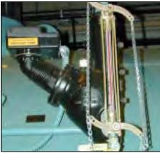
Figure 2-5. Low Water Cut Off
