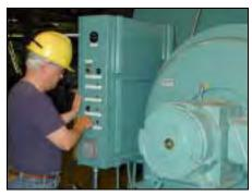
Figure 5-2 Burner Control Panel
