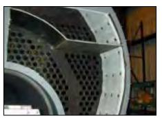
Figure 1-6 Front Baffle Between 3rd and 4th Gas Pass
