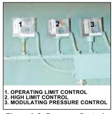
Figure 1-9 Pressure Controls
