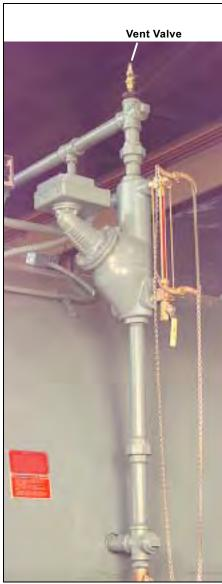
Figure 2-11. Vent Valve on Water Column
