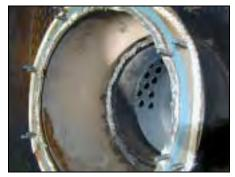
Figure 2-6 Fireside Inspection and Cleaning (Wet-Back Boiler, Rear Door Open)
