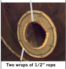
Figure 2-14 Rope Gasket on Rear Access Way
