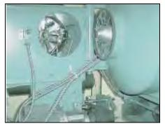
Figure 5-11 Burner Swung Out for Service
