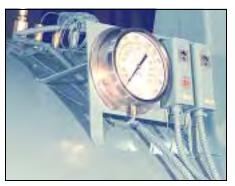
Figure 1-13 Hot Water Temperature Controls
