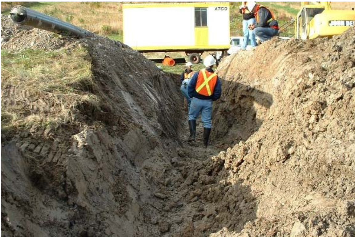
Figure 5.53: Excavated trench showing no sloughing prior to rainfall at test site
