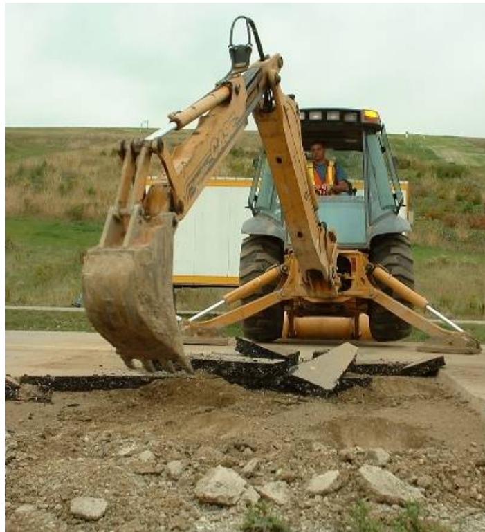
Figure 5.27: Saw cutting of pavement with circular saw
