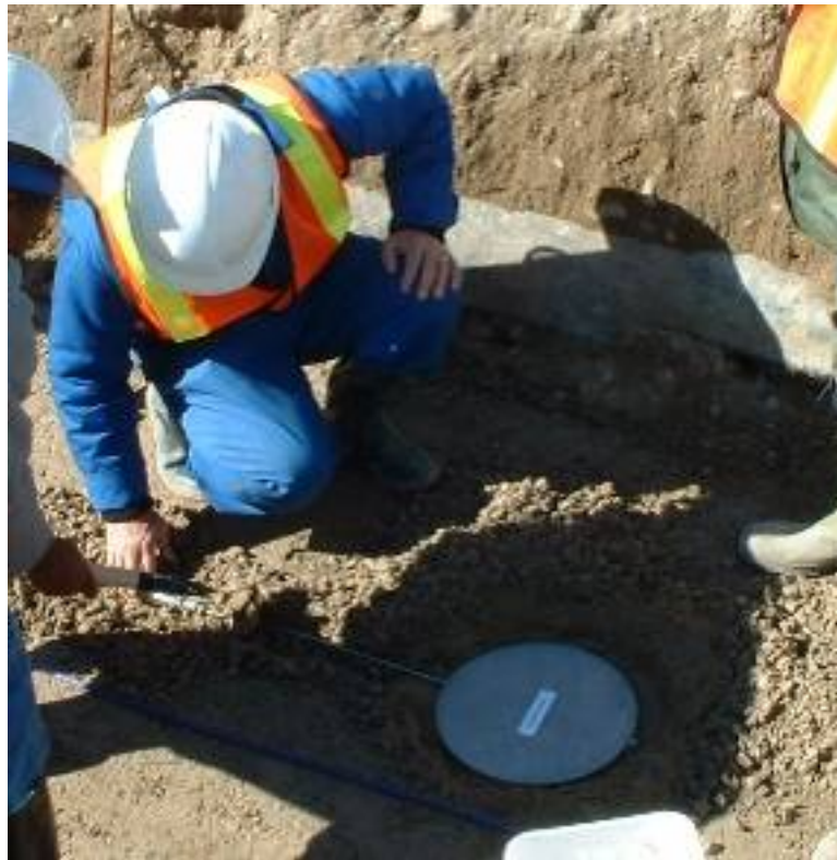
Figure 5.16: Installation of hydraulic total earth pressure cell
