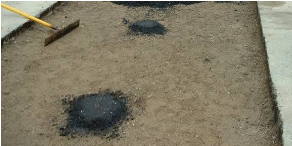
Figure 5.15: Asphalt strain gauge covered with HMA
