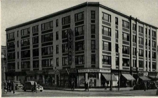
Dauphin Office Building, Harrisburg, Pa. T. A. Bell & Son, Calking Contractors.
