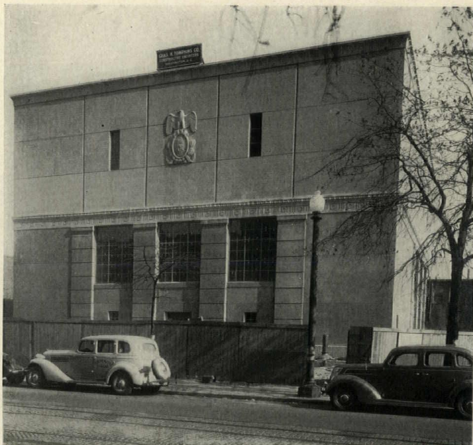
Two views, front and back, of the Warehouse of the Government Printing Office in Washington, for the design of which the Supervising Architect of the Treasury gets credit
