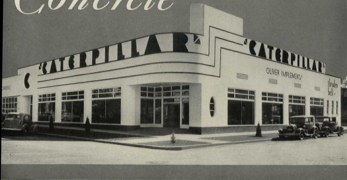
Braden-Bell Building at Walla Walla, Washington. Harold E. Crawford, architect. E. Mardis, contractor. Exterior concrete walls finished with cement paint. Floors, too, are concrete.
