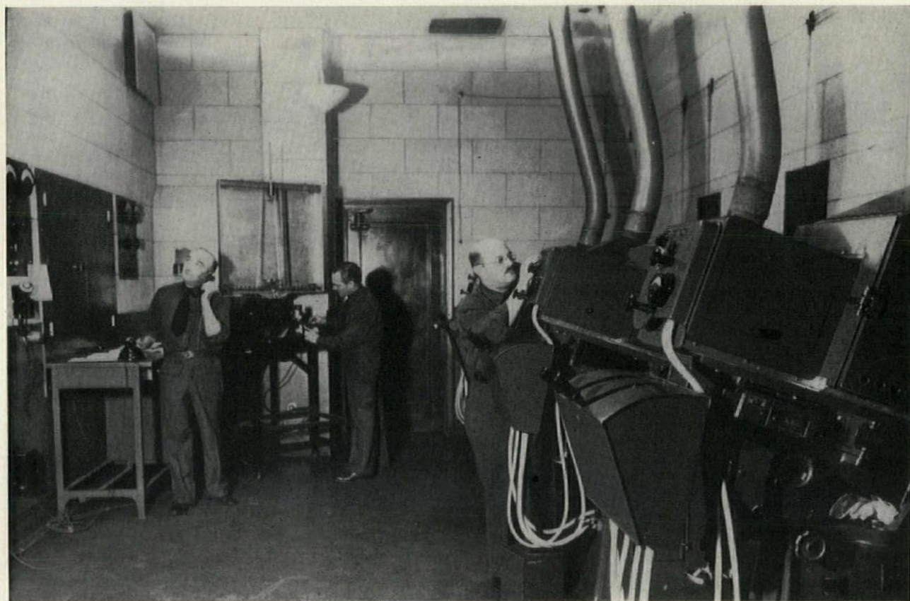
The spacious, airy room from which films are shown at the Radio City Music Hall is far different from the cramped, telephone-booth-size projection rooms of earlier movie theaters. Note the ample ceiling height to insure good ventilation, and the width of room to provide adequate working space behind the projectors. The beam of light, carrying the image of the film, must travel 191 feet to project a picture 23 feet high and 30 feet wide on the screen. The Music Hall screen is the largest ever used in an indoor theater, measuring 40 by 70 feet
