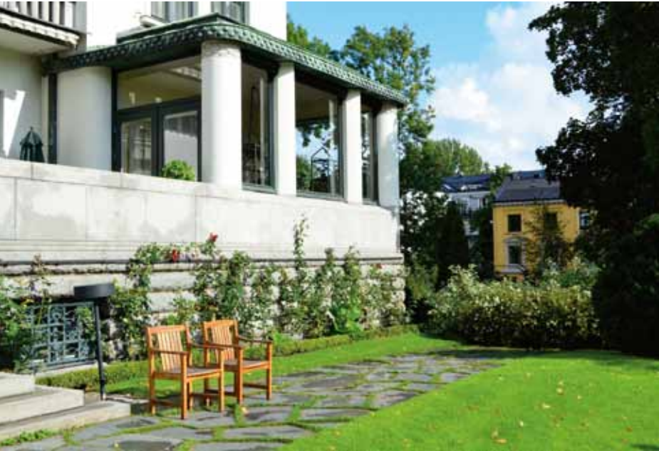
Southern façade with glass-enclosed “winter garden” room that links dining room to rear garden.
