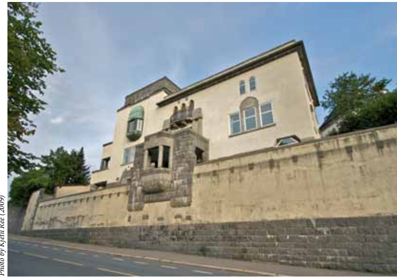
Bryde House at Kristinelundveien 22.
