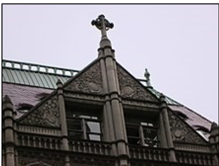
Pignon au sommet de Church Missions House.
