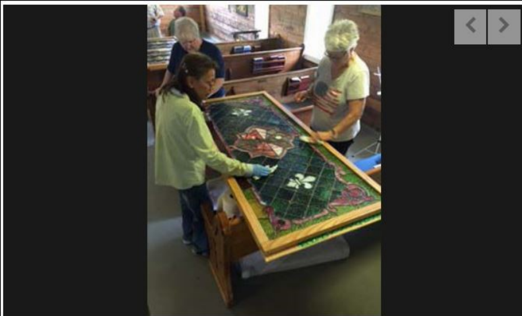
Volunteers from North Carolina prepare the windows to be installed.
