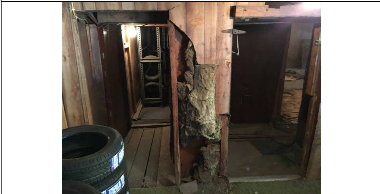
View from loft into Dining Room and Tire Storage 4.
