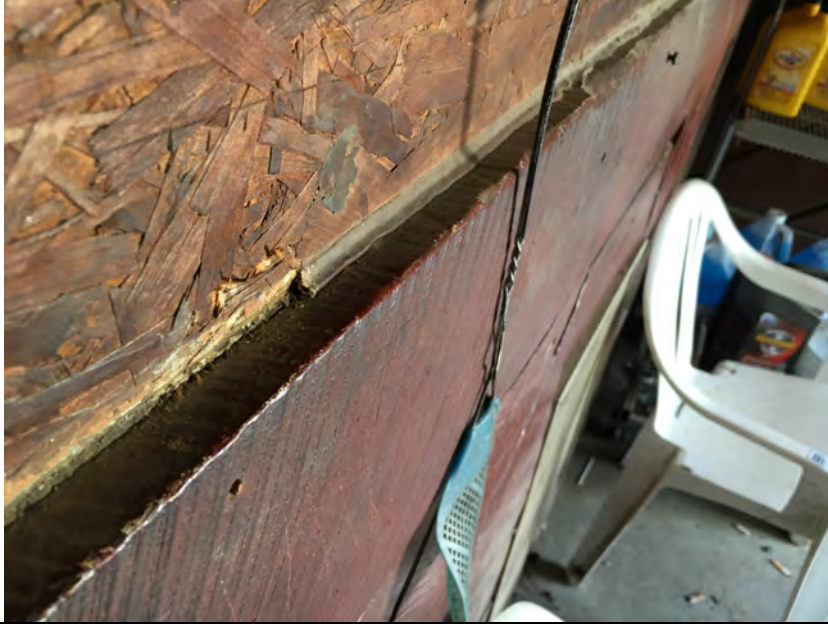
Caulk sealant in Office 1.
