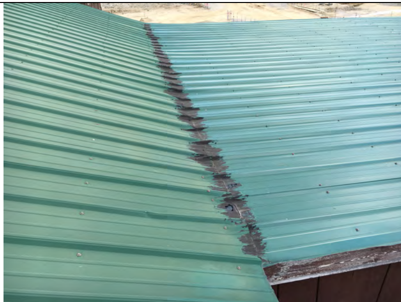
View of roof and roofing mastic. Mastic is non-ACM.
