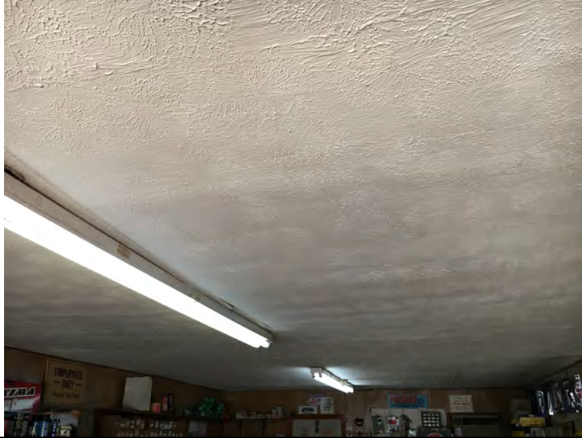
Ceiling texture and gypsum board ceiling in ATV Shop.
