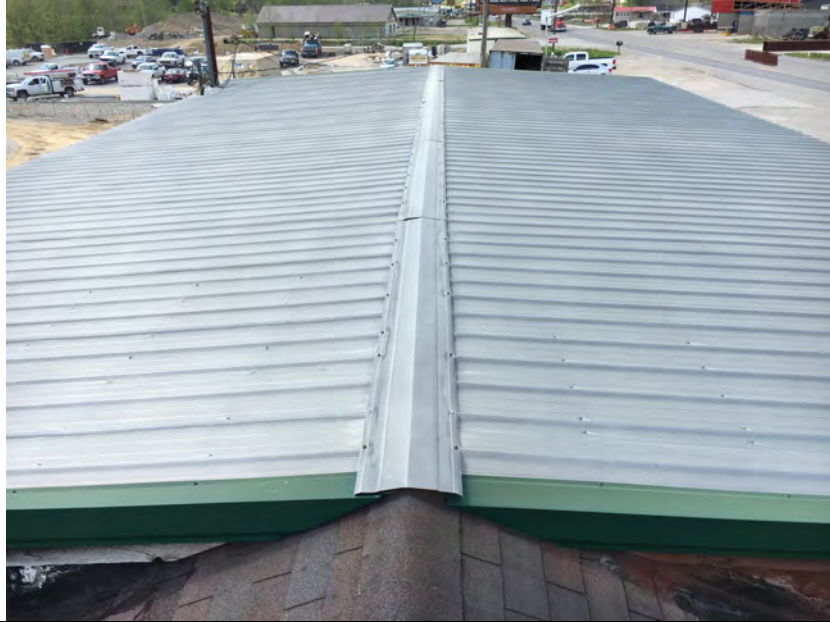
View of anodized metal roof on Subject Property.
