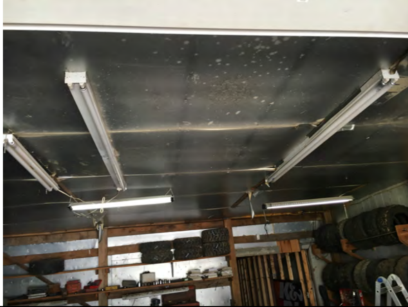
Ceiling of ATV Garage.
