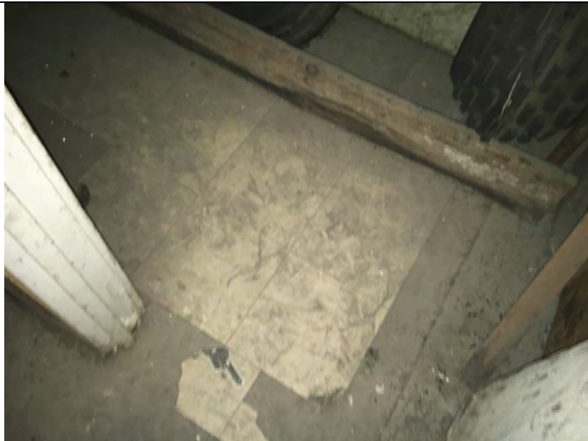
Vinyl Floor tile located in closet. (ACM)
