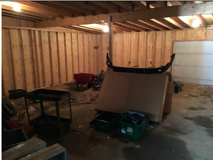
Interior view of Garage 2.
