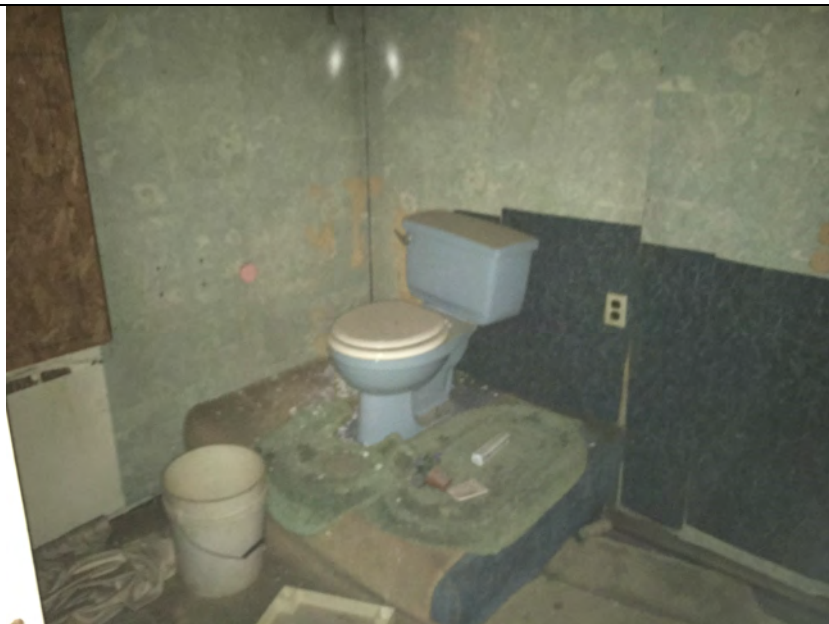
View of Bathroom 2.
