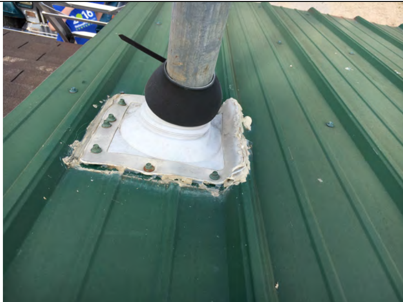
View of caulk on roof penetration.
