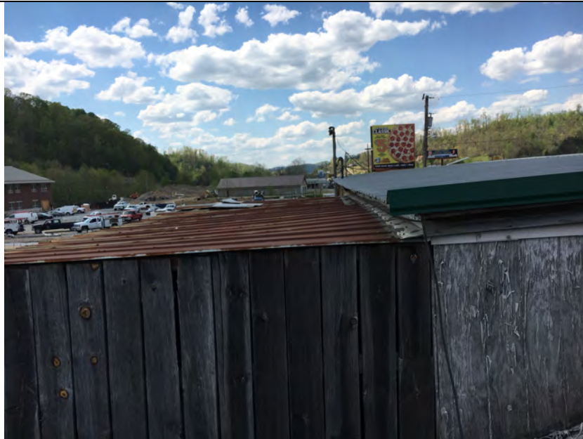
View of roof and roofing mastic. Mastic is ACM.
