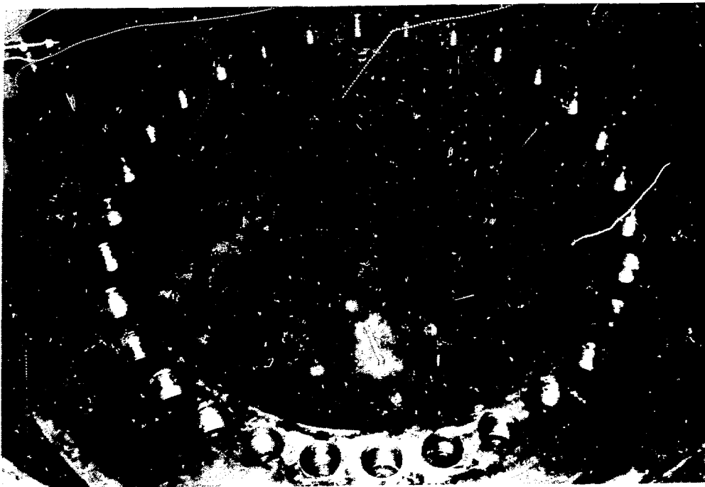
Fig. 6. The main circulating pump case after the decontamination Decontamination Equipment For The Collectors Of The Steam Generator
