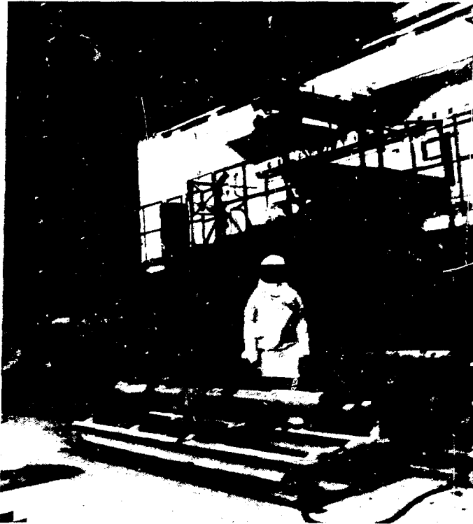
FIGURE 5 RETUBING TOOL CARRIER AT REACTOR FACE
