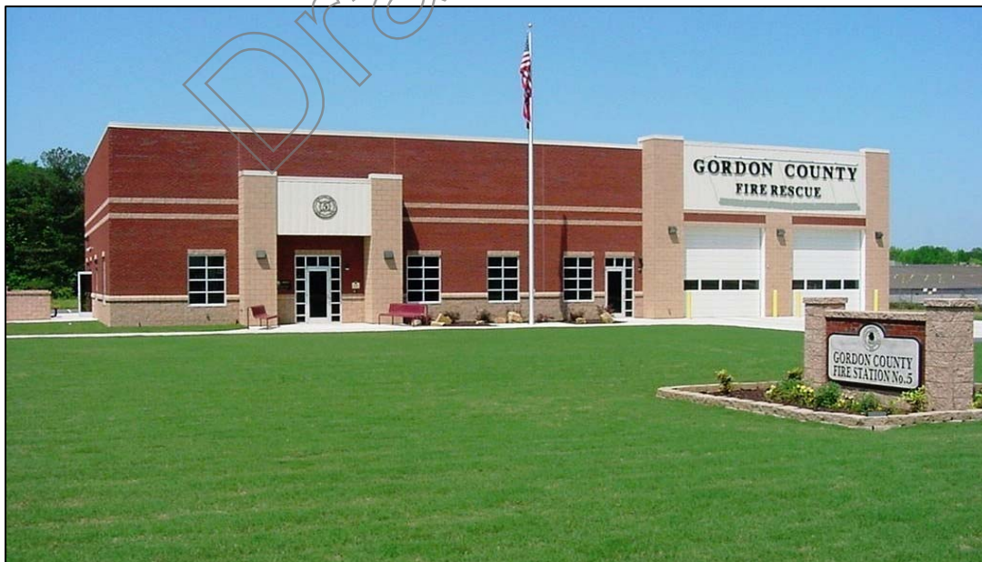
Gordon County Fire Station in Resaca
