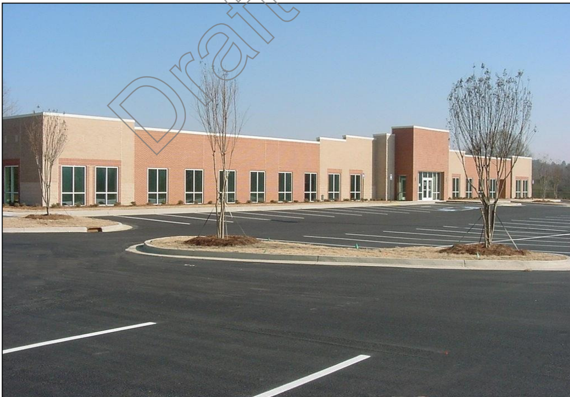
New Gordon County DFACS Building
