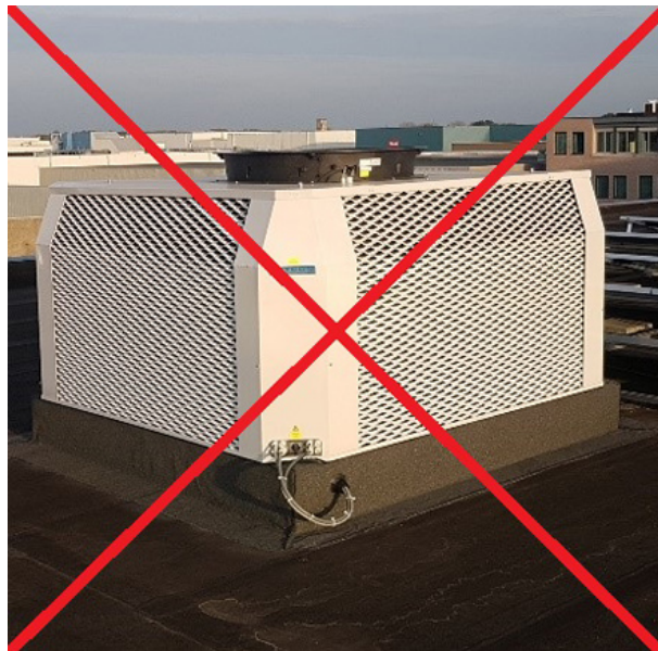
Wrong installation example (poor accessibility of the drain valve)
