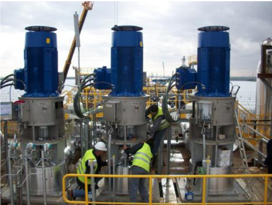
Figure 1 Modern oil platform
