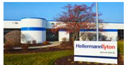
Offices and Manufacturing 87th Street, Milwaukee, WI
