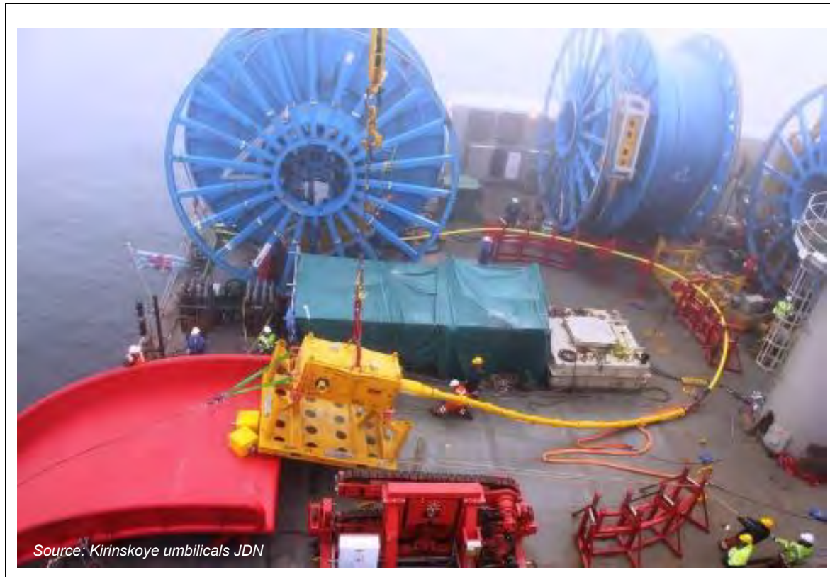
Photo 3.3. Umbilical being driven to unspool over the side of an installation vessel
