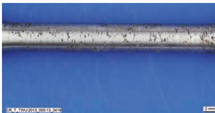
Stainless steel with pitting corrosion, e.g. A4 material used in a road tunnel
