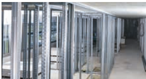
Drywall tracks to concrete and steel
