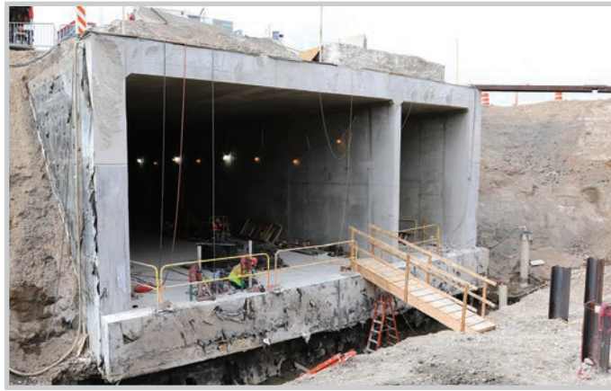
North Tunnel Opening - June 2018
