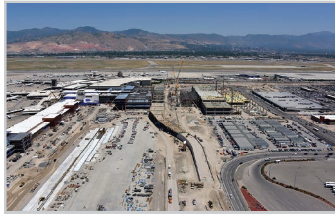
Terminal Area Looking West - June 2018
