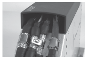
Shield connection with clip and metal cable ties
