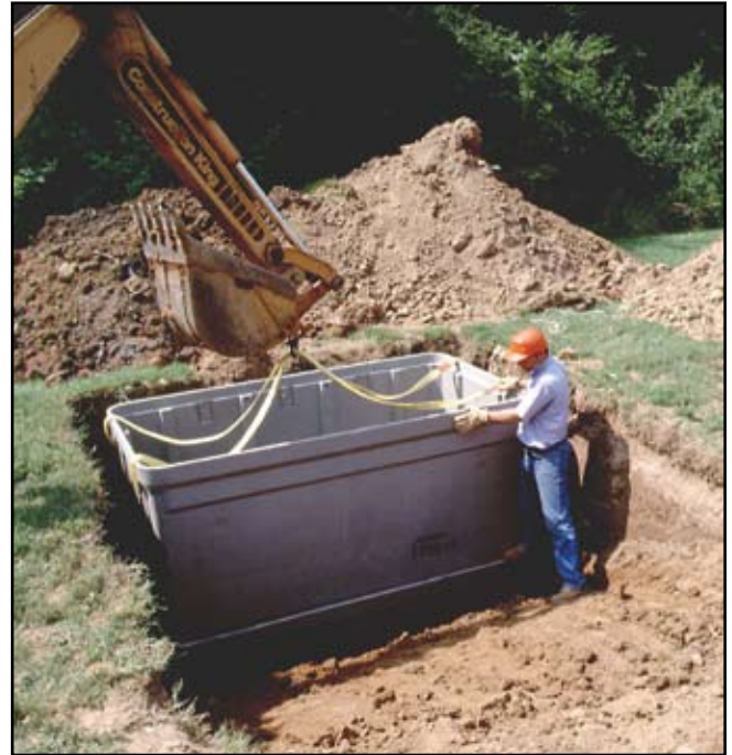
The strong polymer concrete construction allows QUAZITE® enclosures to be stacked for even greater depths.
