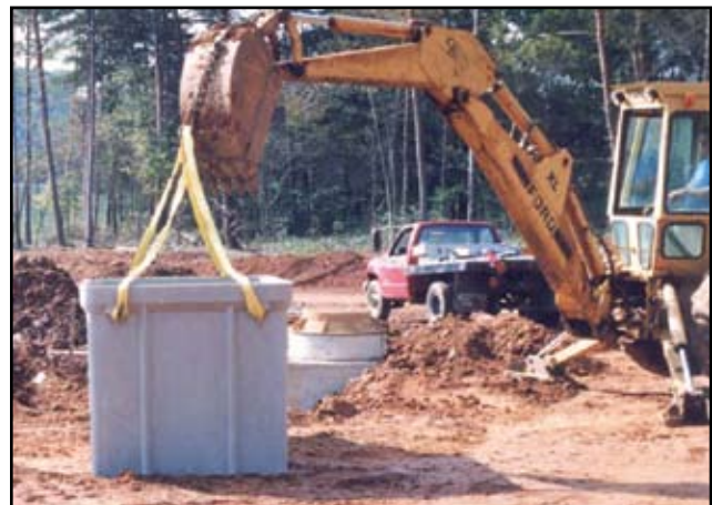
Lift and position enclosure with backhoe (4.03).
