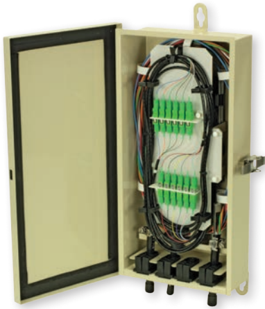
LL-500 with interconnect kit installed
