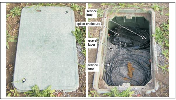
Figure 67: Ground level buried vault closed and open
