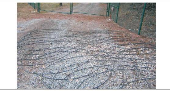
Figure 56 Laying cable in a figure-8 pattern
