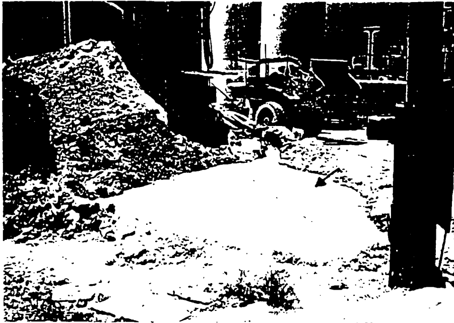
Figure 3 Arrow indicates re-liquidified lime which will be loaded onto a tank truck and used for road stabilization.
