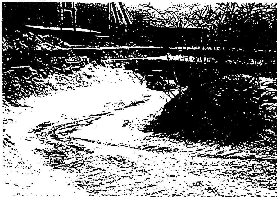
Figure 2 Excavation of solid lime pit.
