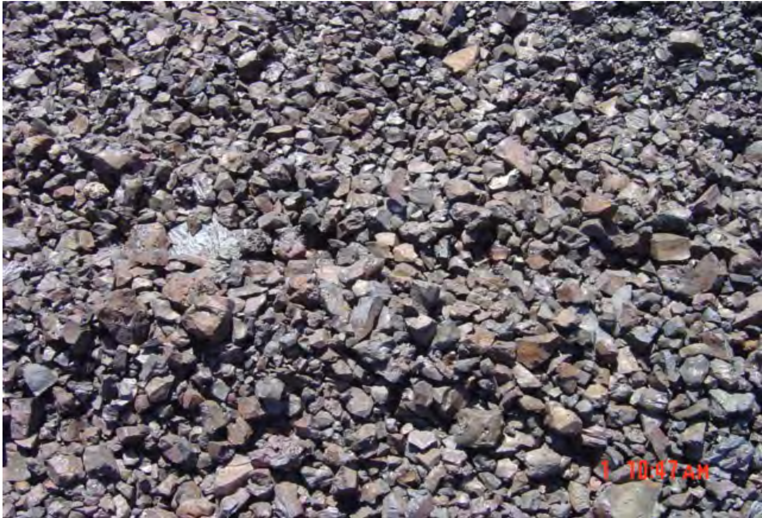
Closer image of crushed furnace slag used for erosion repairs to lower bench near southwest corner of Impoundment AB.
