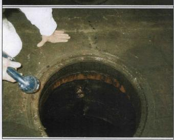
PHOTO 15 Site Name: M&H Zinc TDD#: S05-0808-001 Location: Lassalle, Illinois Date: 10/1508 Direction: Down Photographer: T. Koach Description: Oil material inside manhole; note oil on two pipes leading into manhole.
