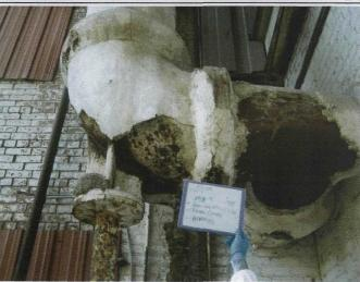
PHOTO 6 Site Name: M&H Zinc TDD#: S05-0808-001 Location: Lassalle, Illinois Date: 08/26/08 Direction: Up Photographer: T. Koach Description: Sample MH-9, pipe insulation on ESE side of Rolling Mill.
