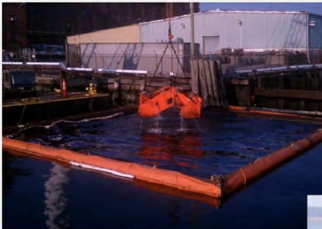
Cable Operated Environmental Clamshell Bucket and Dredge Cell Courtesy of CableArm Environmental Systems @ www.cablearm.com
