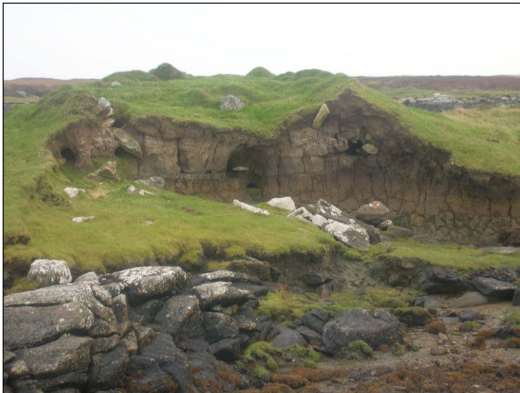
Plate 2. Peat erosion at Àird nan Laogh (cell 8, Map 2)
