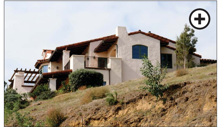
A home in the Alta Vista neighborhood is set into hillside to create a “low profile”. (28.2, 28.3, 28.4, 29.1, 29.2)
