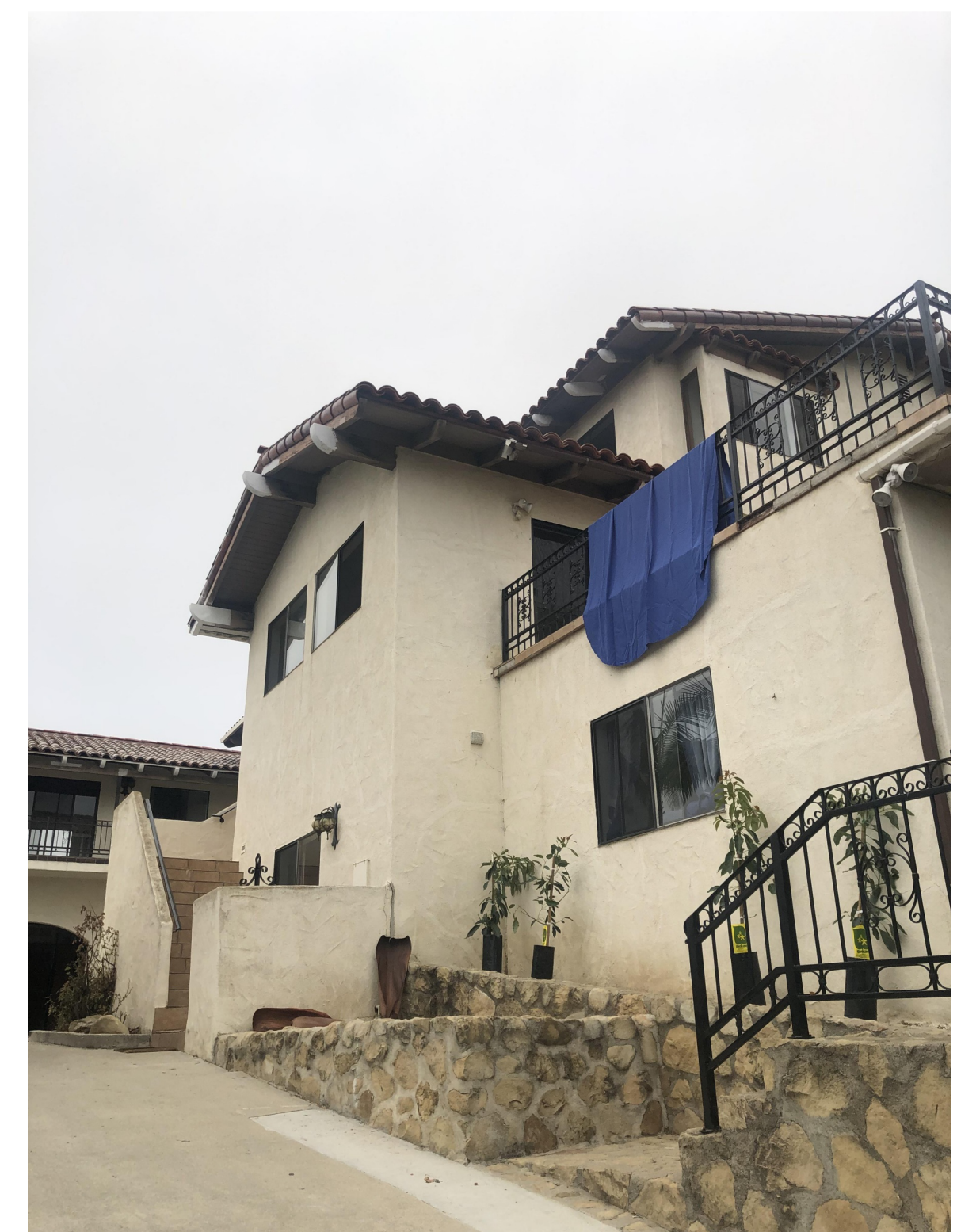
VIEW FROM MID DRIVEWAY
