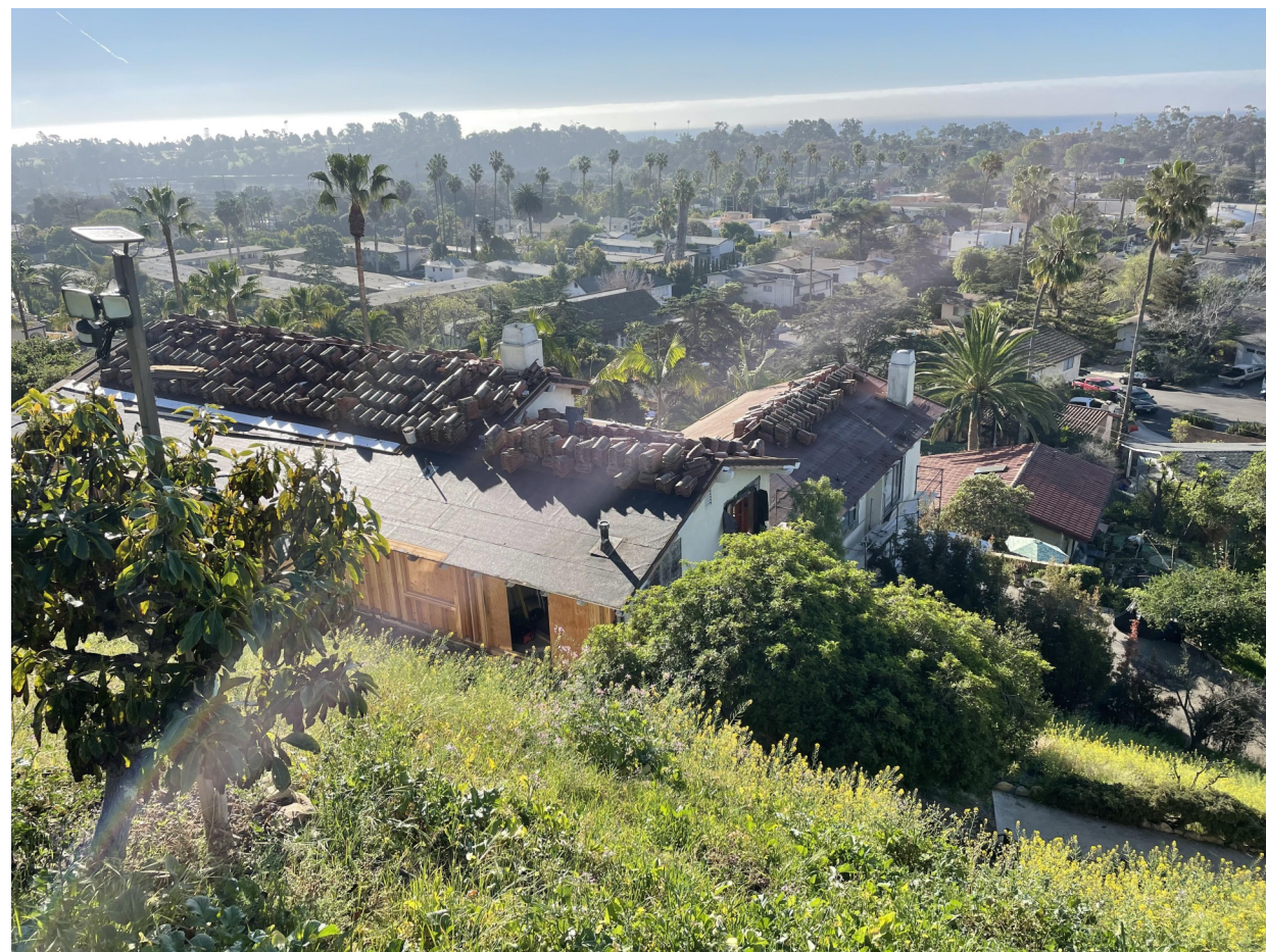
UPPER HILLSIDE VIEW - NORTH
