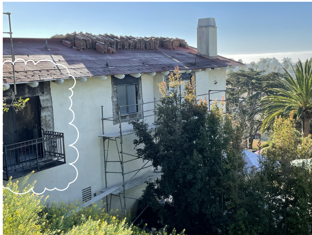
EXISTING BALCONY - WEST ELEVATION
