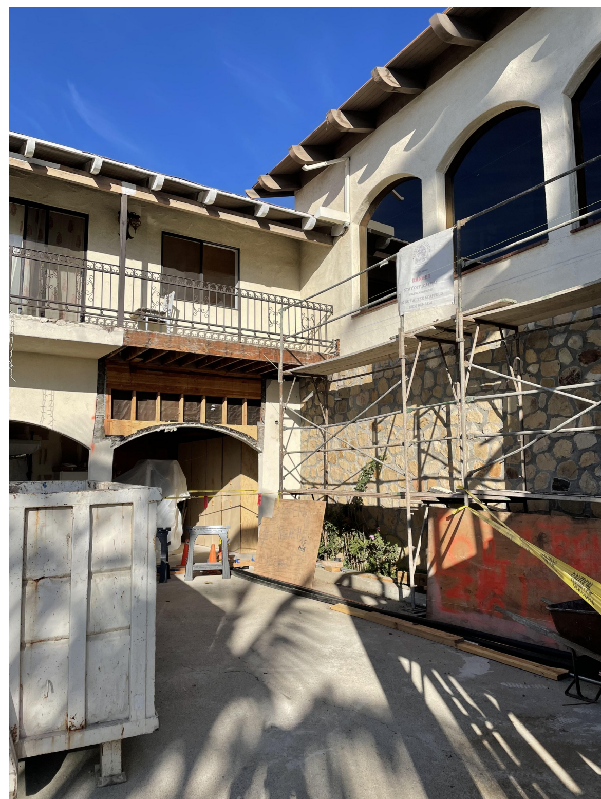
VIEW FROM ENTRY STEPS
