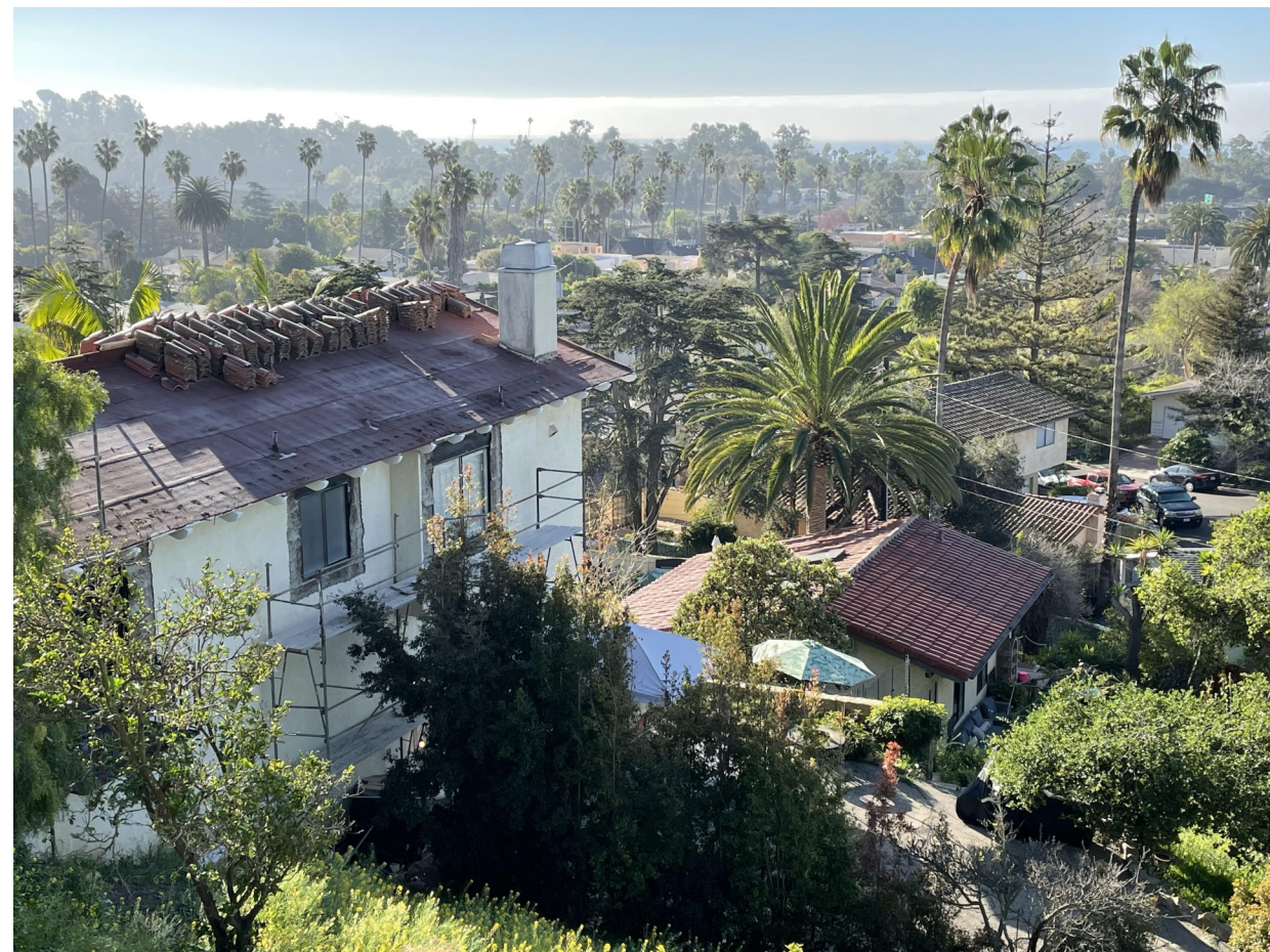
MID HILLSIDE VIEW - NORTH
