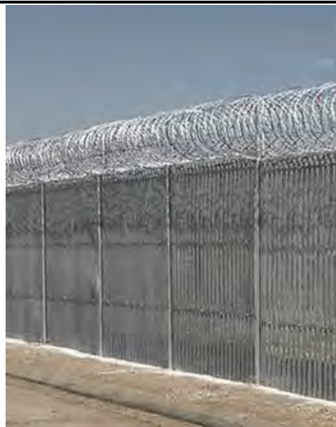
Figure 3.15 Illustration of the fencing that will be used ('Clear Vu', 3m high)
