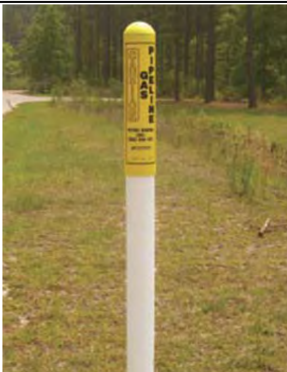
Figure 3.31 Example of a marker indicating pipeline below ground
