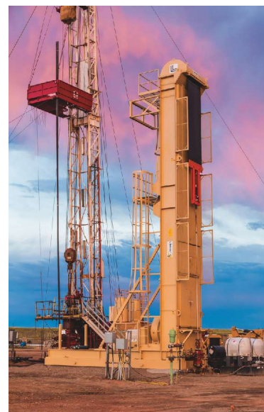
The XL Long Stroke Pumping Unit was installed in the Bakken on a highly deviated well application to help reduce overall rod cycles and transition from the first to the second form of lift in the life of the well. (Source: Dover Artificial Lift)
