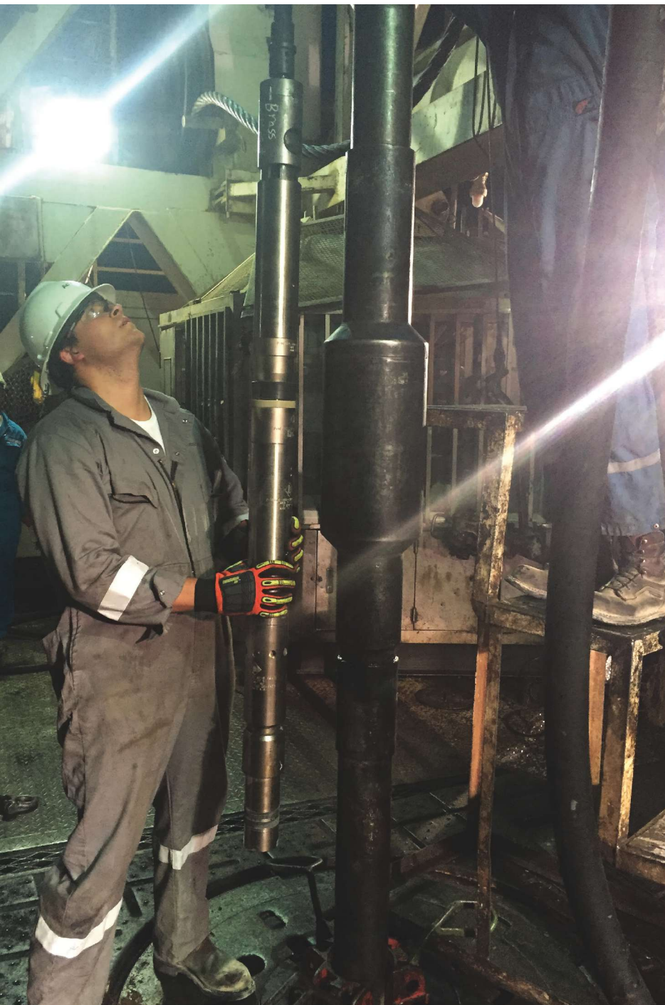
A rig worker runs the AccessESP tool into a well. (Source: AccessESP)
