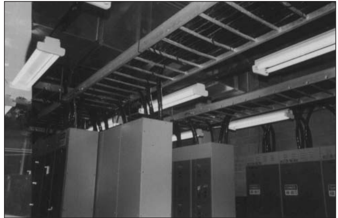
Cables Exiting 480 Volt Outdoor Switchgear and Entering Cable Tray System (Cable fittings with clamping glands are required to prevent moisture flow into equipment due to the cable's overhead entry into the switchgear enclosure).
