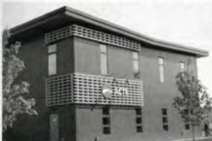
Addison County Transit Resource Office & Bus Facility Completed 2013
