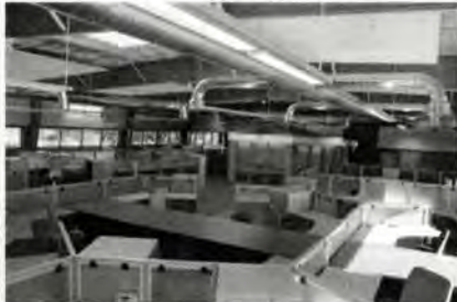
VELCO Warehouse to Office Conversion Completed 2013
