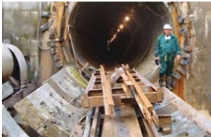
CAPTION: Workers laying a cable line
