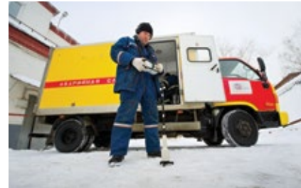
CAPTION: The testing and measurement service of JSC “MOESK” branch – Moscow Cable Networks checking the operation of cable equipment
