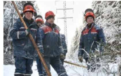
CAPTION: Workers restoring power following the freezing rain
