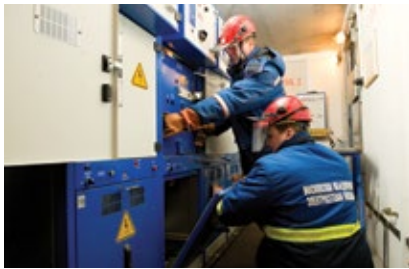
CAPTION: Installation of 20 kV equipment
