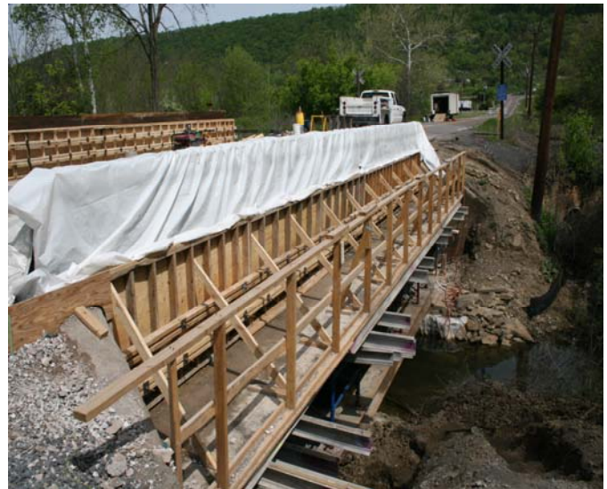
Figure 6: Extensive Formwork along Beam 1
