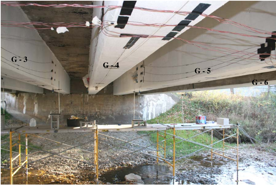
Figure 45: Overall Test Setup
