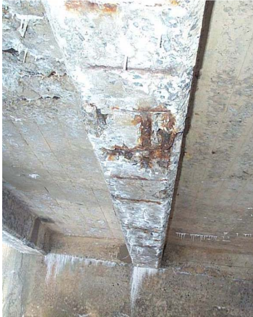
Photo on left: NCHRP Report 514, an example of a T-beam suitable for FRP-wrap technology
