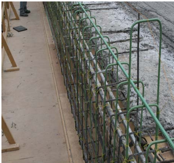
Figure 1: Complete Removal of Concrete from Beam 6, Exposing the Reinforcement
