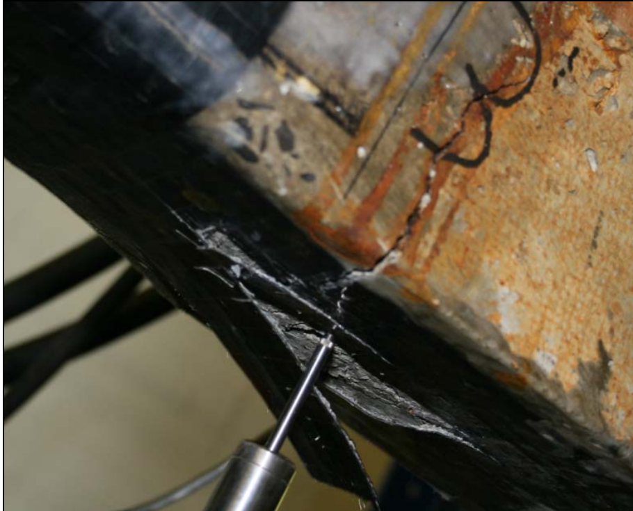
Figure 85: FRP rupture on PMC-repaired beam G-8
