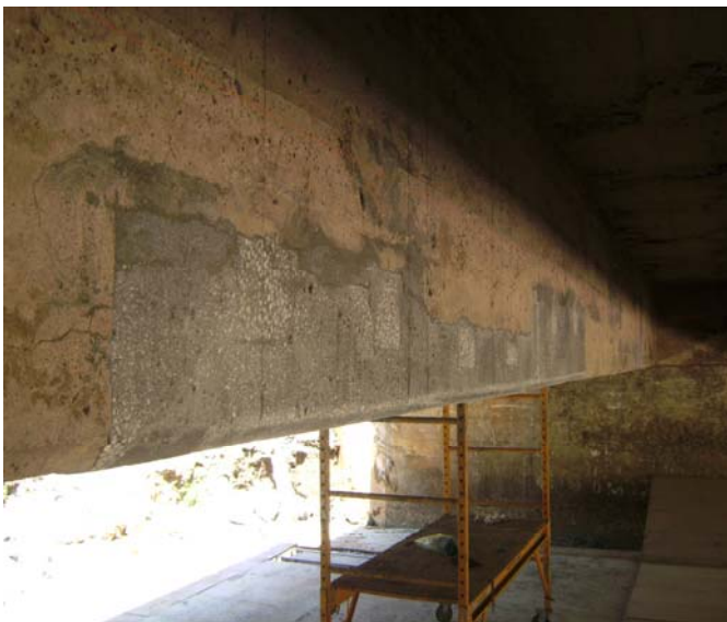
Figure 7: Beam 4 after Patch Repair
