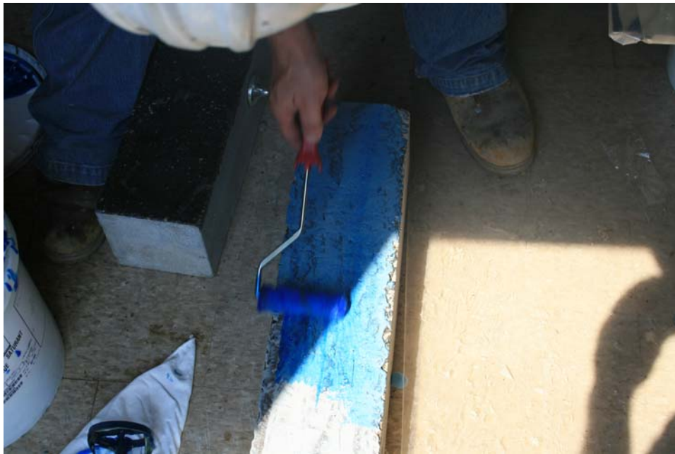
Figure 13: Resin Applied to Test Prism Prior to FRP Installation
