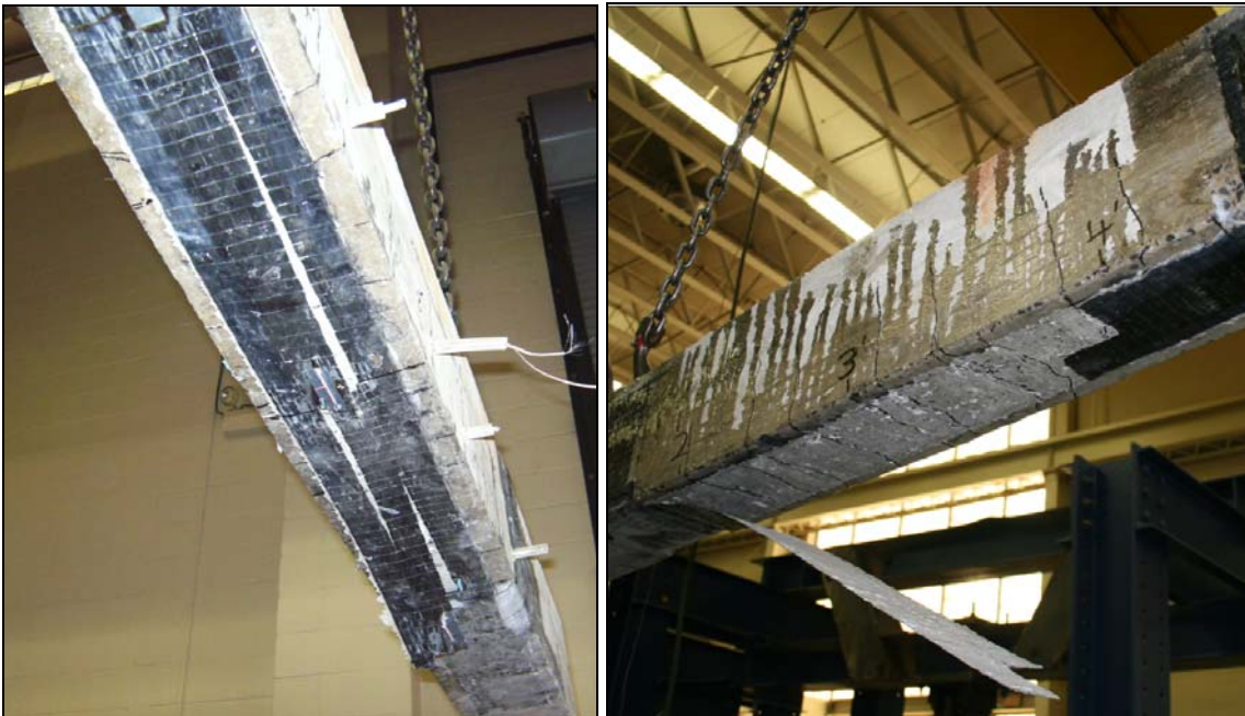
Figure 118: Photos of fatigued Part II beams repaired using Wrapping Scheme 2 after failure
