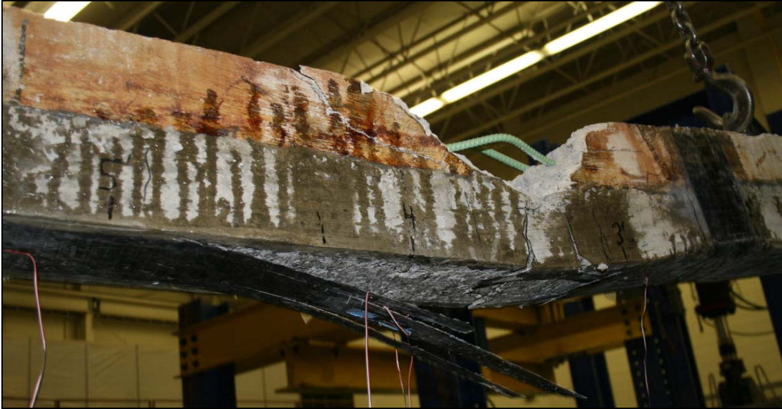
Figure 84: FRP Rupture on PMC-repaired beam G-5
