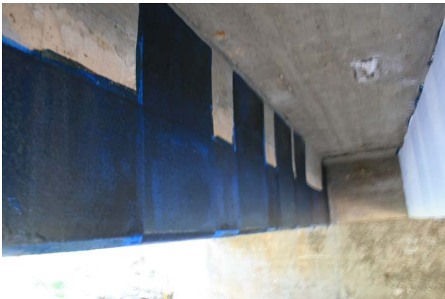
Figure 10: FRP U-Wrap along Beam 5
