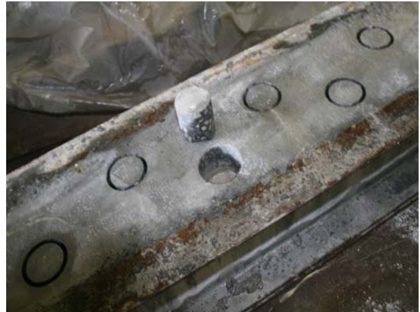
Figure 19: Cores Drilled for Pull-Off
