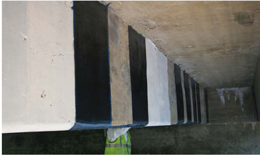
Figure 11: FRP Shear Reinforcement on Beam 2
