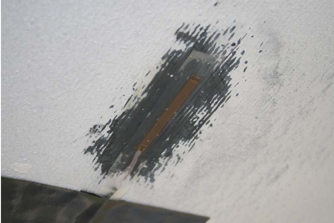
Figure 41: Gage on Flexural FRP
