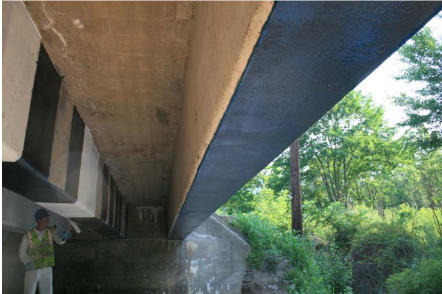
Figure 9: Flexural FRP Reinforcement along the Bottom of Beam 1
