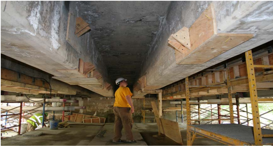
Figure 4: Formwork for Patch Repairs along Beams 3 and 4
