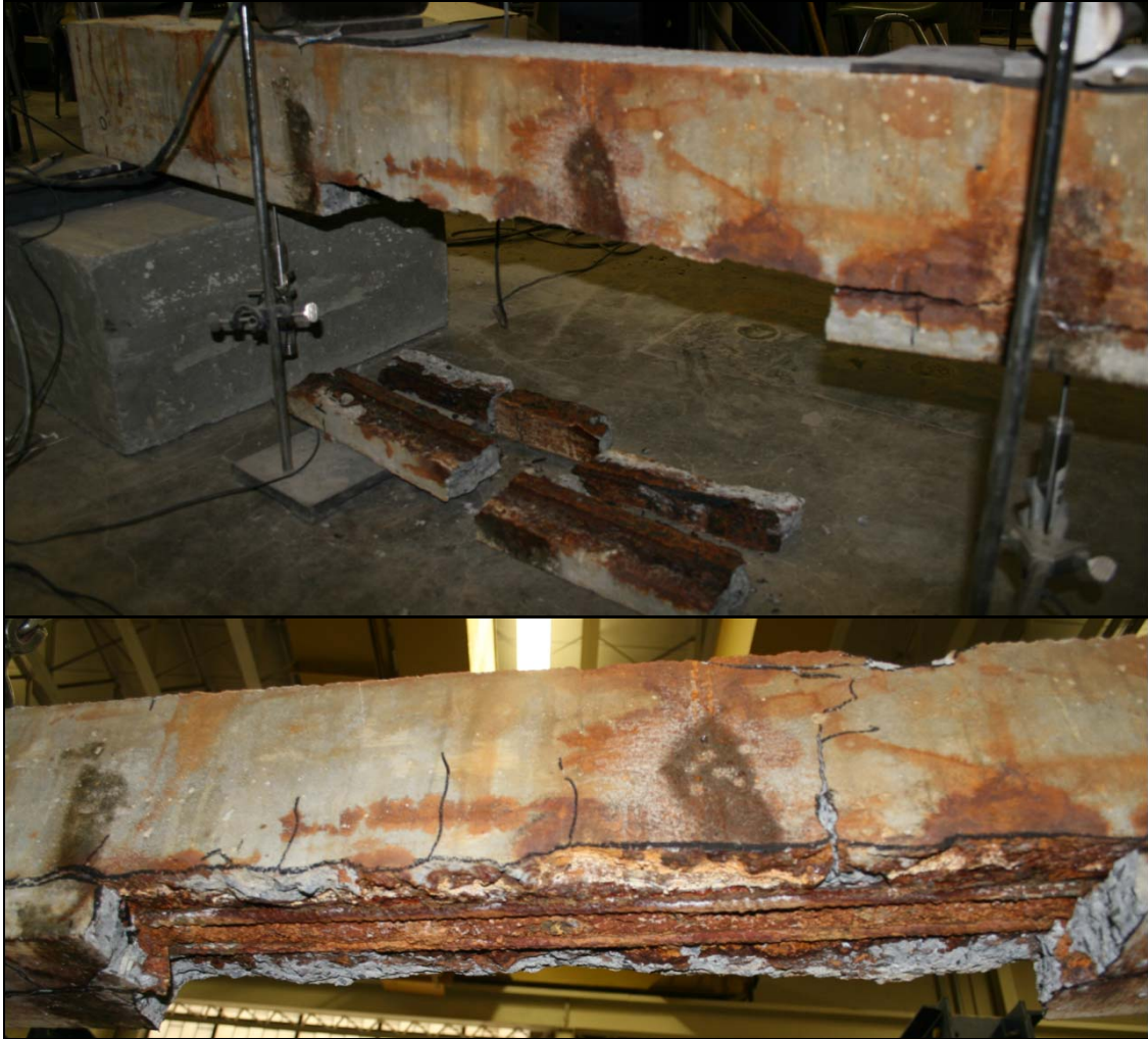
Figure 121: Failure of Beam II-4
