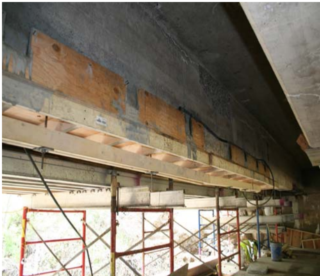
Figure 5: Formwork along Beam 5
