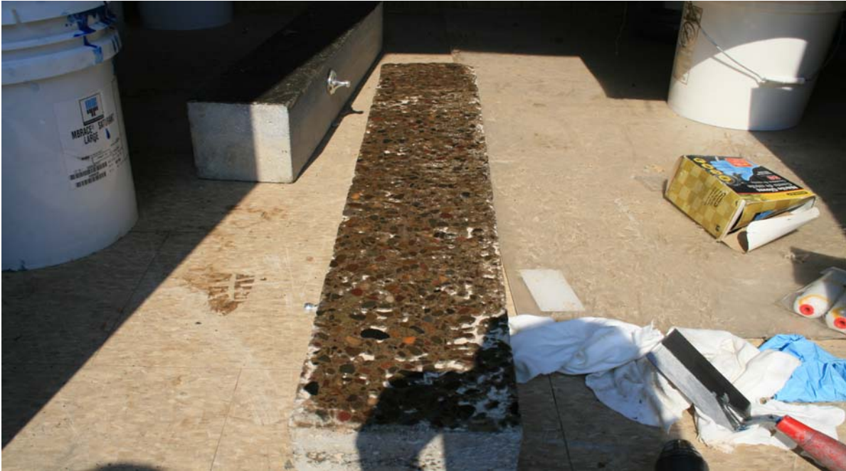
Figure 12: Test Prism Coated with Primer Prior to FRP Installation
