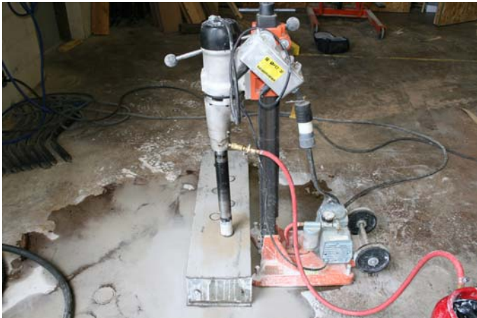
Figure 18: Core Drill Set-up used for Concrete
