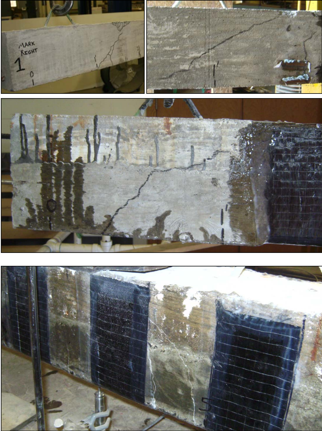
Figure 123: Typical shear flexure cracks observed on Part II beams
