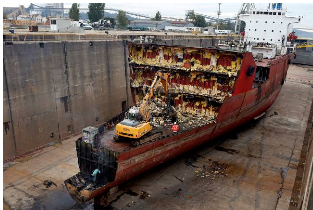
Bassens, Matterhorn being dismantled in drydock © R Escher
