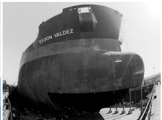
Under repair at San Diego © Aukevisser.nl
