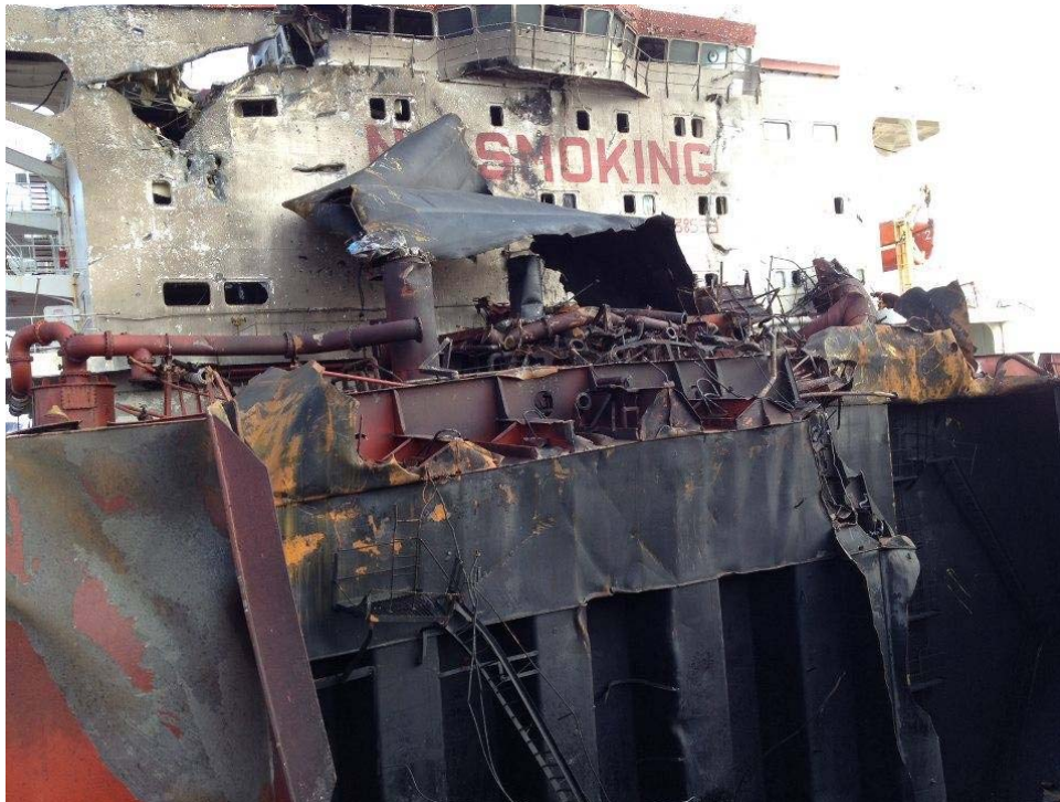
No smoking, welding OK © Cargolaw
