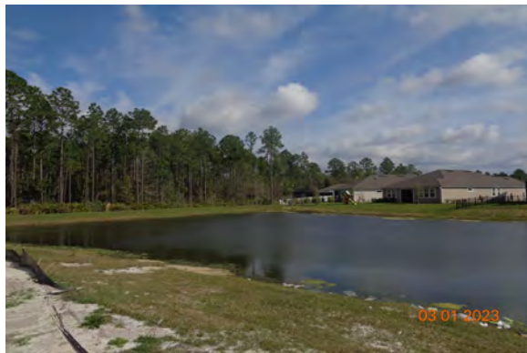
Pond MM: Previous treatment was effective.
