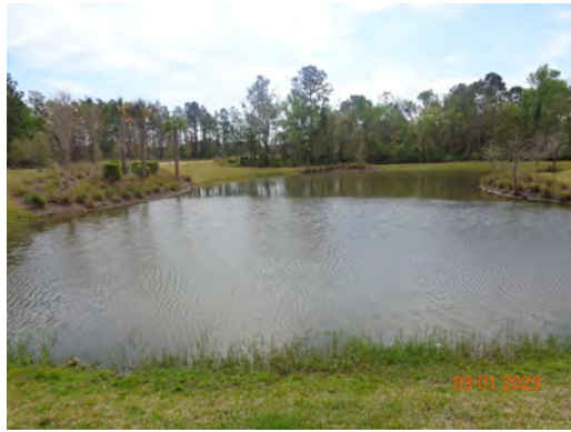
Pond WW: Pond in good condition, treated perimeter weeds.
