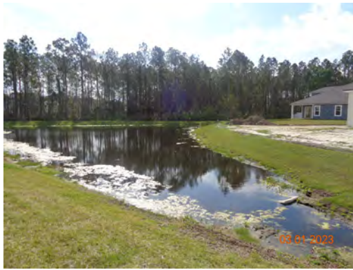
Pond GG: Pond in good condition, previous treatment was effective.
