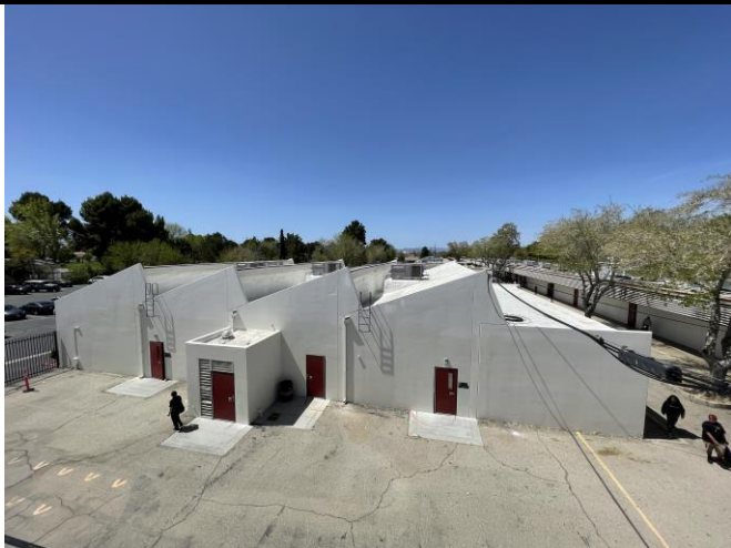
Photo 5: Building 31 (typical of Buildings 31, 32 and 33)
