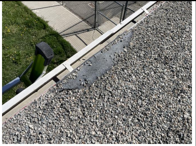
Photo 8: ACM roof mastic on Building 32
