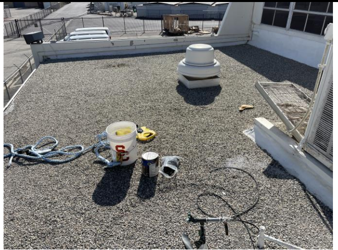
Photo 6: Flat roof on Building 33
