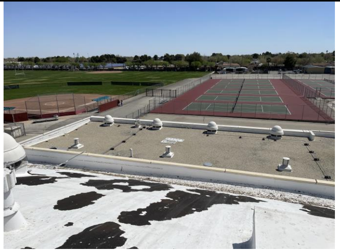
Photo 4: Girls Gym lower roof
