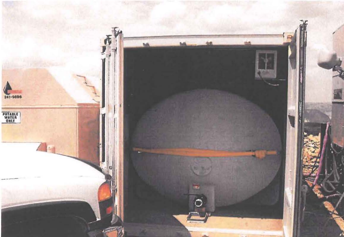
Photo 6. Sealed 4,000 Gallon Wastewater Tank in Heated Enclosure.
