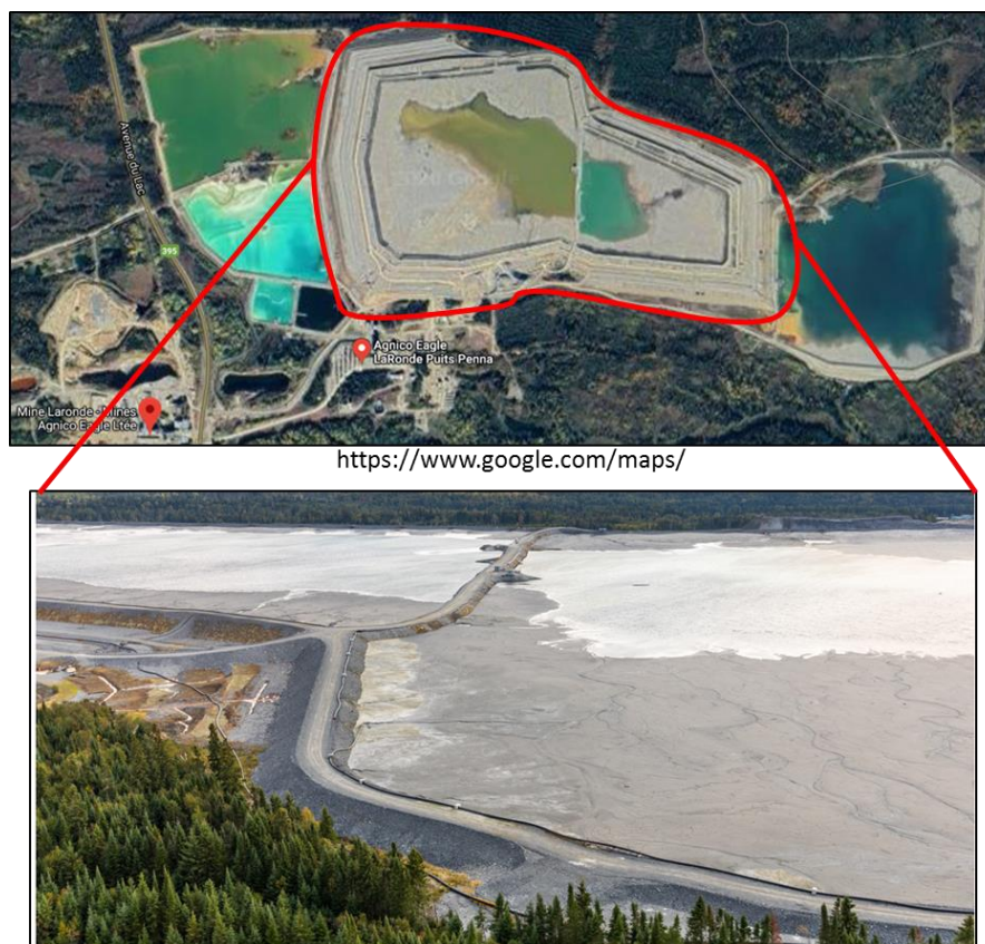
Figure 6.1 LaRonde tailings storage facility.
