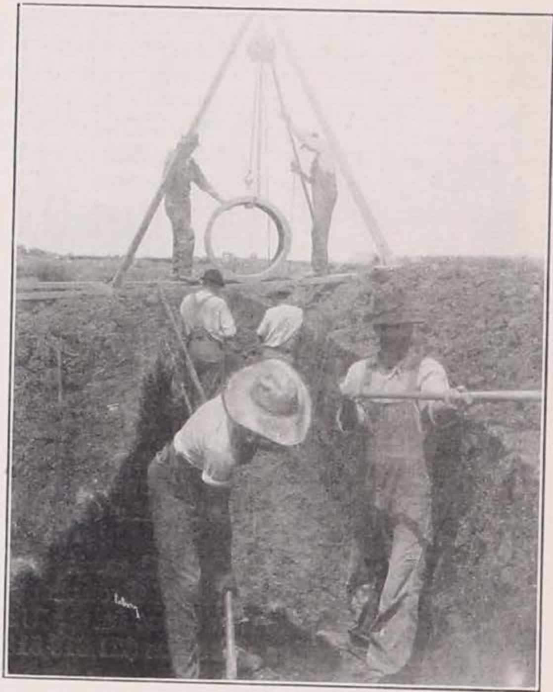
Fig. 2. The Construction of a 36 Inch Tile Drain in Boone County, Iowa.
