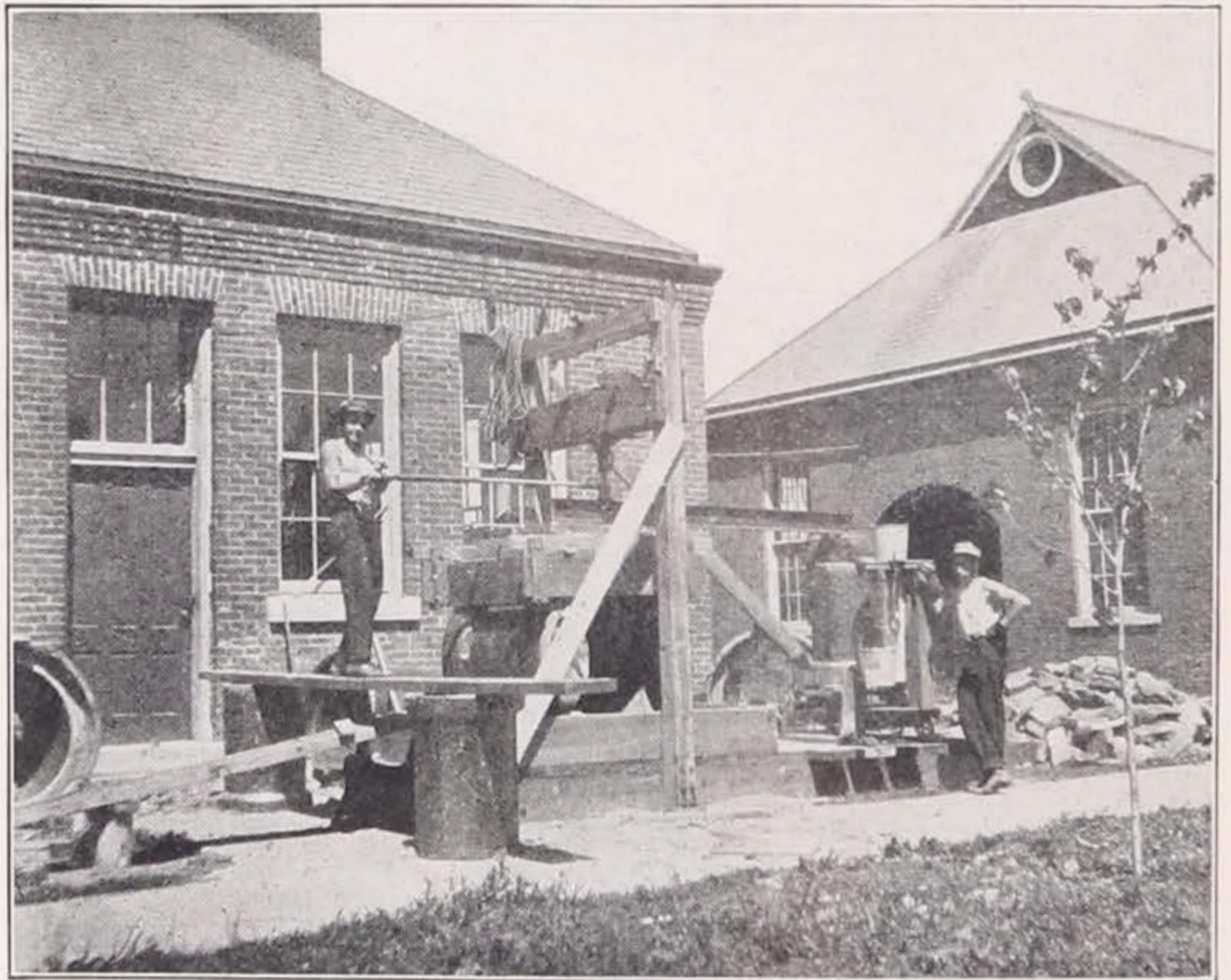
Fig. 27. Several Hundred Dollars Worth of Vitrified Clay Sewer Pipe Free from One Factory, Broken in Tests.
