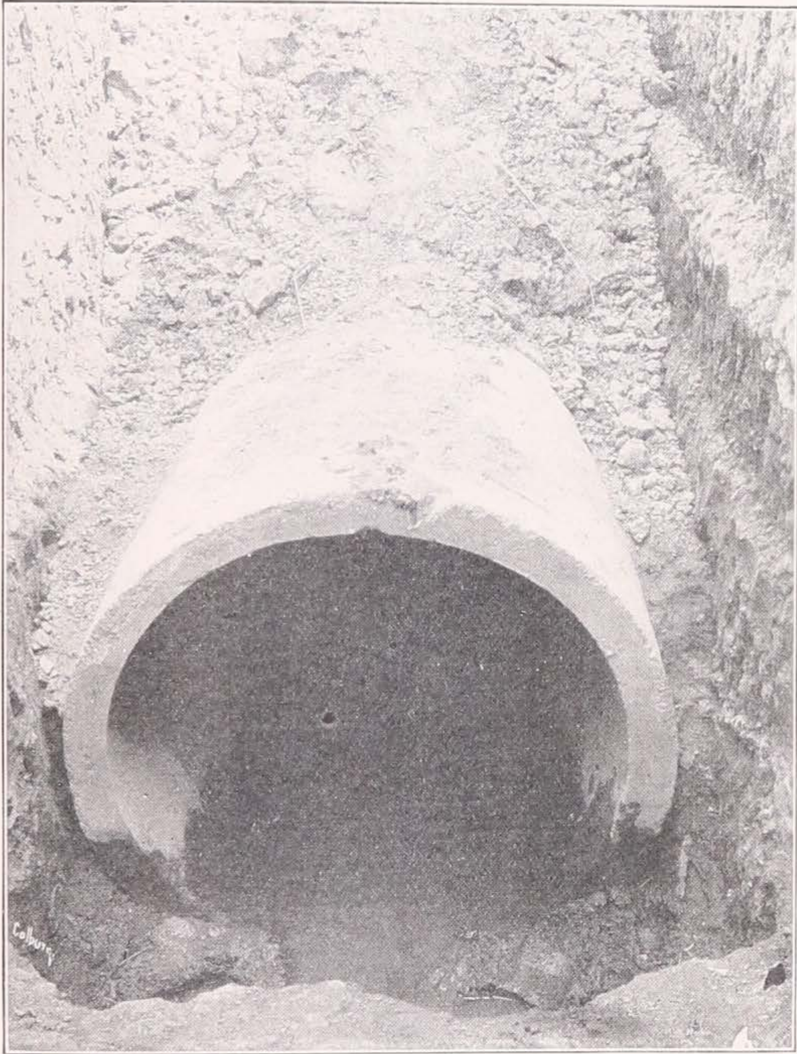
Fig. 23. Photograph Showing the very Best Possible Bedding of Pipes in Ditches.
