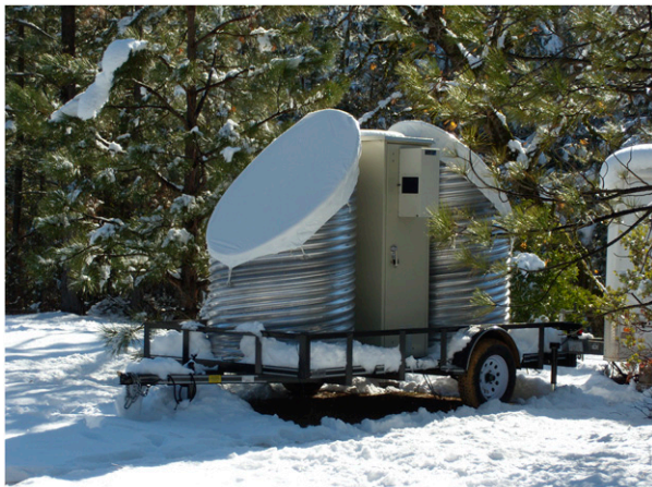
FIG. 1. The Colfax SLR 8 Dec 2009. The TX antenna is in the shroud on the right. The radar electronics are located in the enclosure between the antennas.
