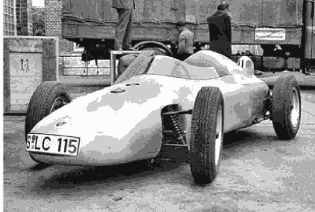
The new 787 – essentially a long-wheelbase version of the updated 718/2. Just two were built (78701 and 78702), the first completed in April. The Porsches looked like bars of soap on wheels compared to the gorgeous 'sharknose' Ferraris, but they certainly got the job done, despite the lack of disc brakes.
