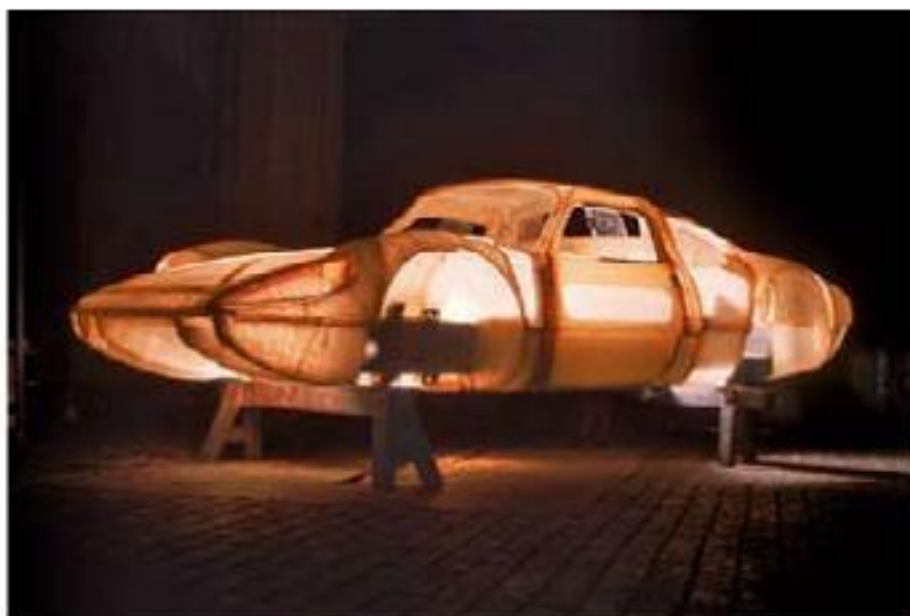
Body production at the Heinkel works in Speyer, and the gossamer-thin finished article. The body was so light that two people could lift it with ease.
