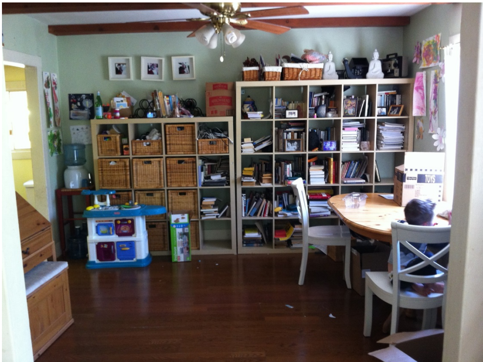
Original ceiling beam work and door frame. Undeterminable directions.
