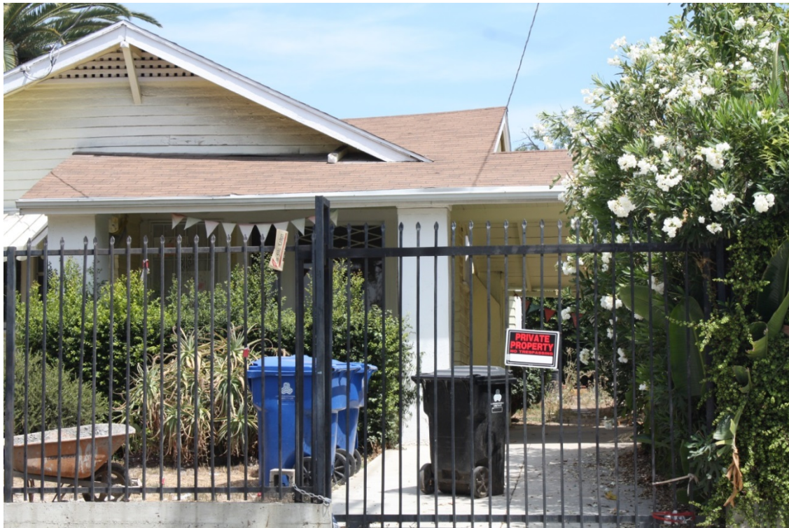
Current condition of 4511 Russell Avenue: August 3, 2015.
