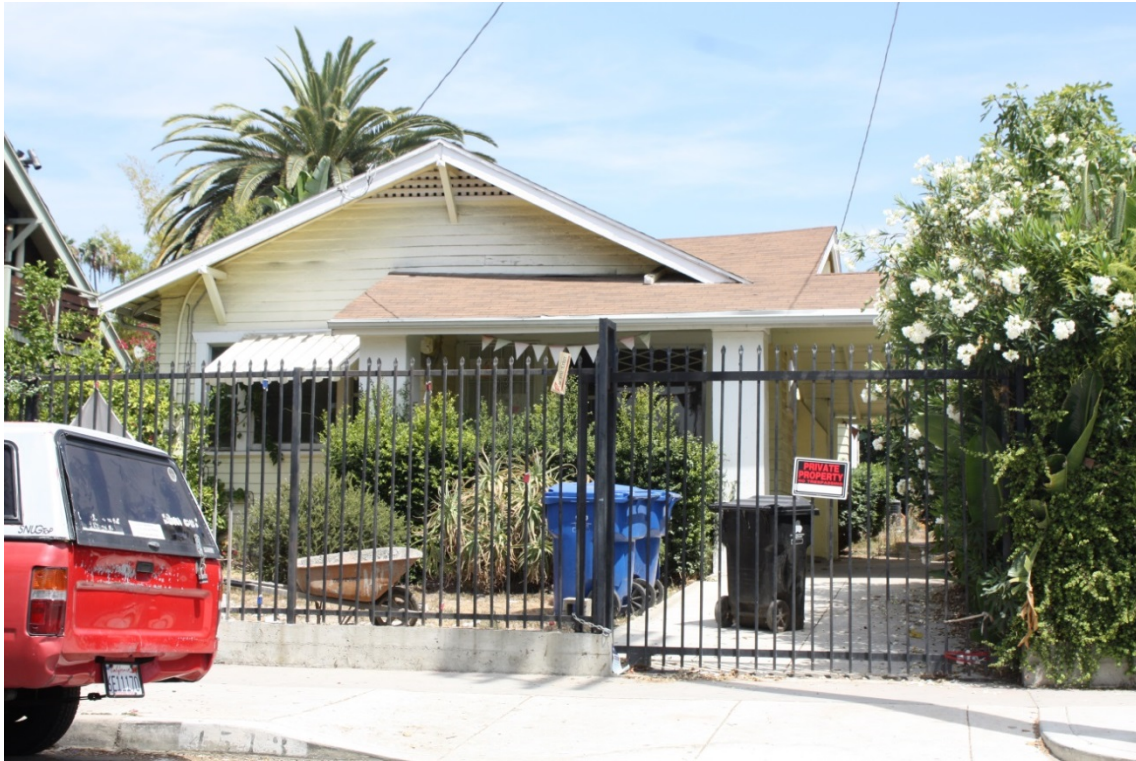
Current condition of 4511 Russell Avenue: August 3, 2015.
