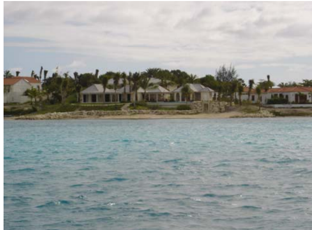
Figure 5.6: Some of the buildings on Long Island within the NEMMA (Espeut photo).
