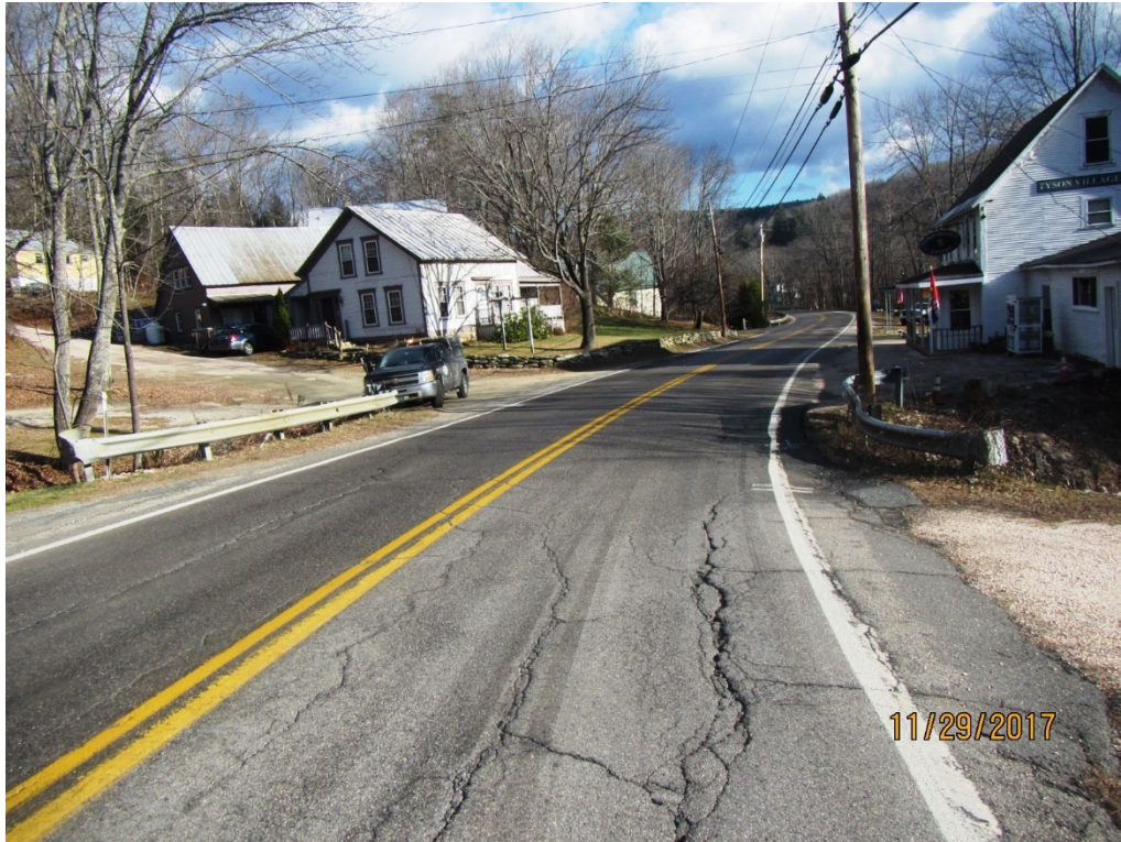
Figure 3.1: Overhead utilities above culvert crossing VT RT 100. [Inspection photo dated 2017]
