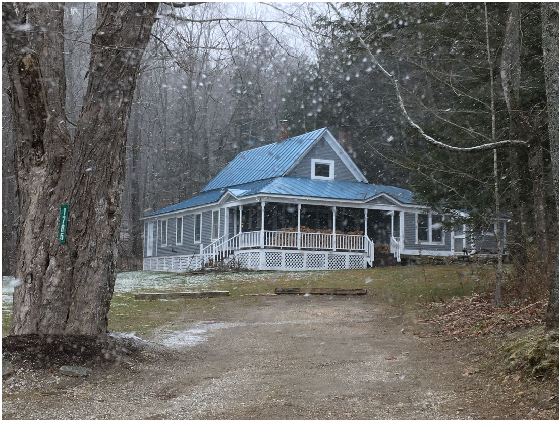
Figure 5. SR-listed house at 1785 VT-100 in Ludlow. SR survey No. 1410-121.
