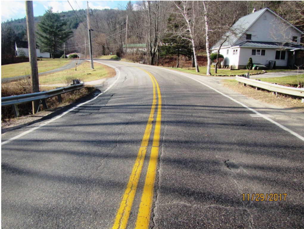
Picture 1: Looking South over Bridge 102
