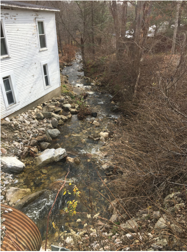
Picture 4: Looking Downstream from Bridge 102
