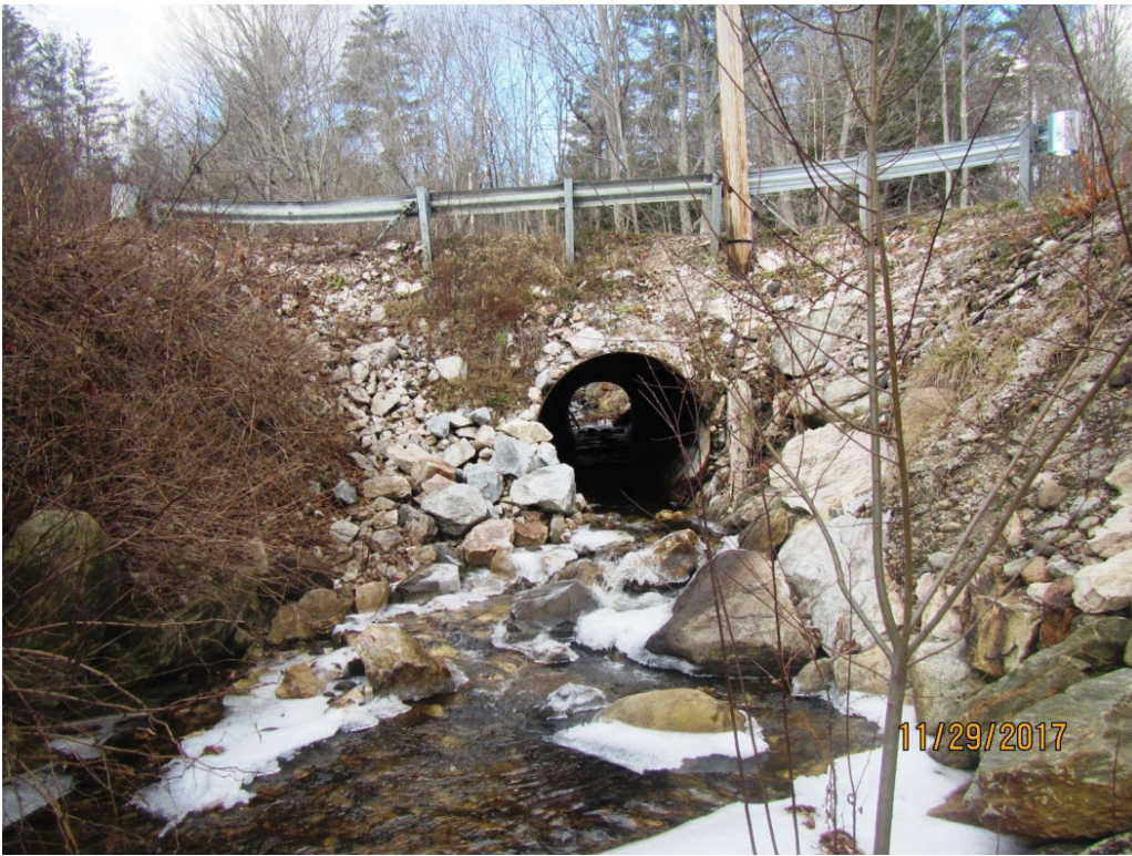
Picture 7: Culvert Outlet
