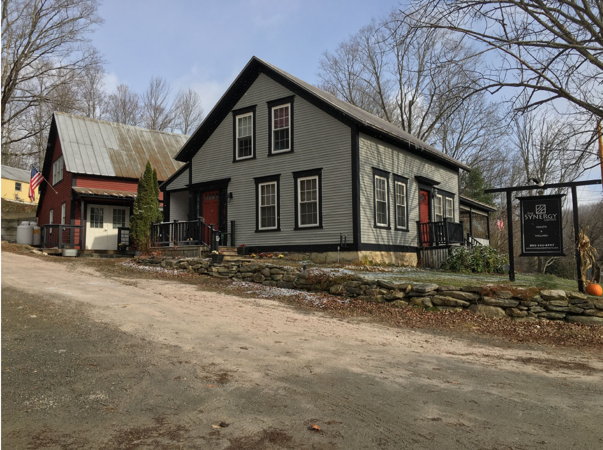
Figure 8. Former Ephraim T. Holt House, c. 1865. SR survey No. 1410-122.
