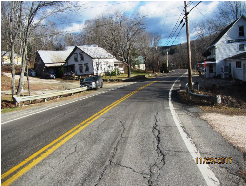
Picture 2: Looking North over Bridge 102
