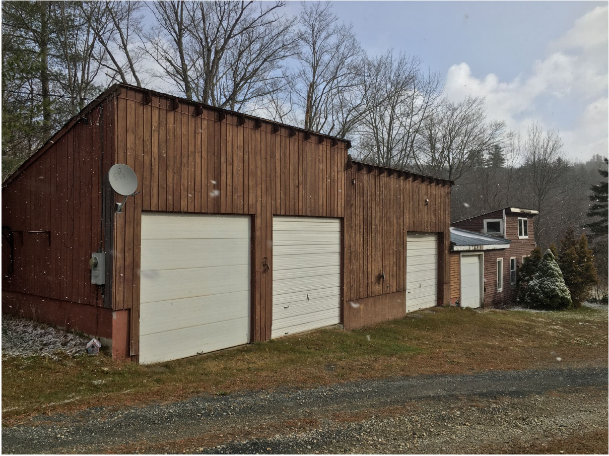
Figure 7. Ineligible building at outlet.
