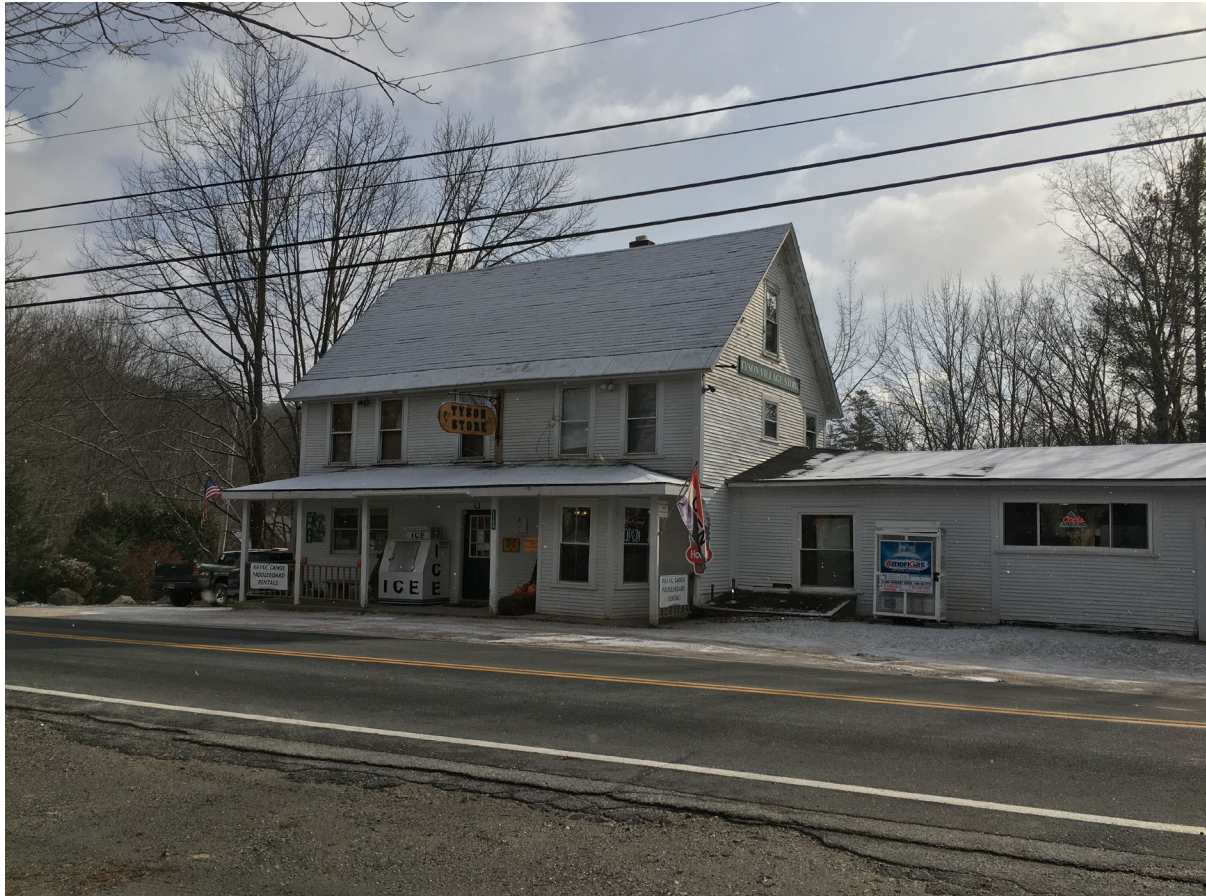
Figure 6. SR-listed Tyron Store. SR survey No. 1410-120.
