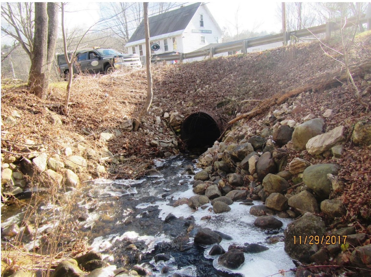
Figure 4. Bridge No. 102 with Tyson Store in background.
