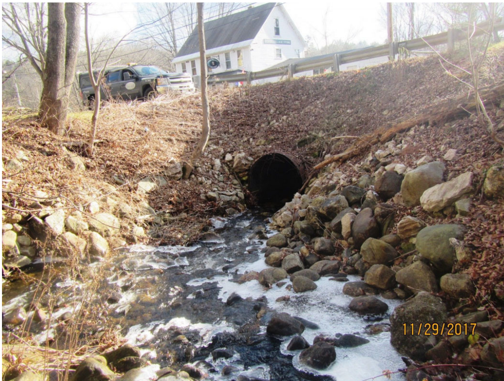
Picture 6: Culvert Inlet
