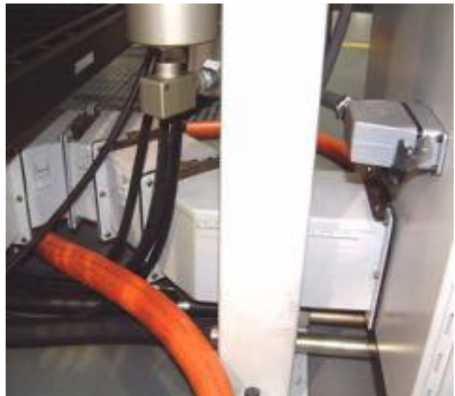
Machine Base Connections
