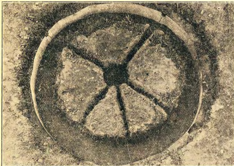
Fig. 2—Installation of the earth electrode.
