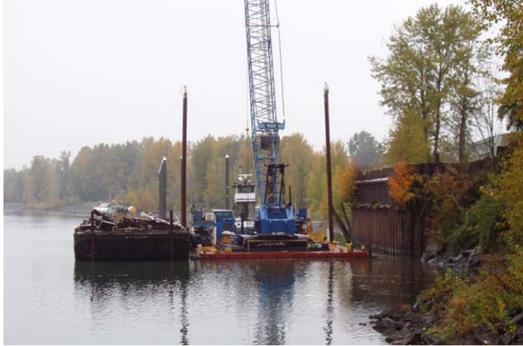
Figure 6: Waterfront Construction at Oregon City
