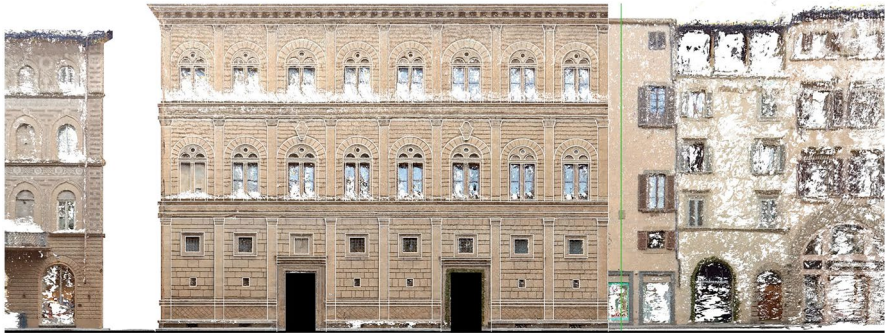
Façade Reconstruction 8-bays
