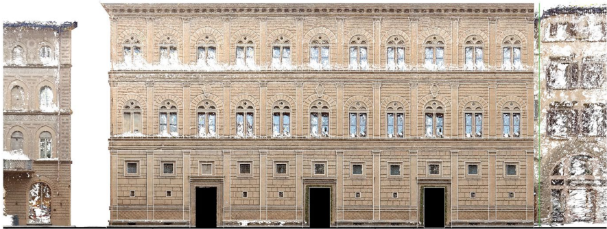
Façade Reconstruction 11-bays
