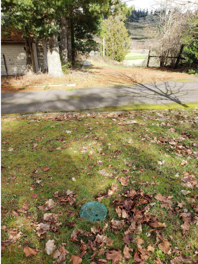
Fig. 3: Location of existing 6 inch cleanout leading to the sewer pump vault station. The existing cleanout will be removed, and replaced with a shallow concrete manhole.
