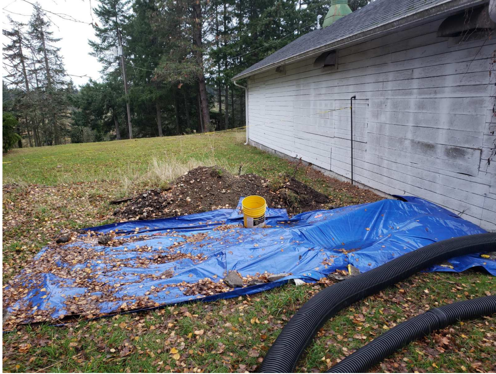
Fig. 1: Current condition of area behind lab.
