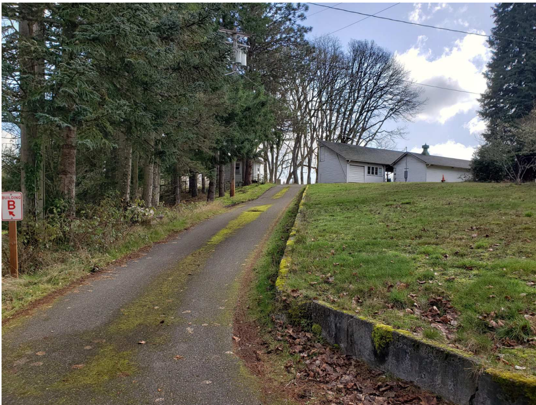
Fig. 4: Lab located at the top of the hill on the right. New sewer line will come out of the rear of the building, and will be placed in the grass and connect to the new shallow concrete manhole.
