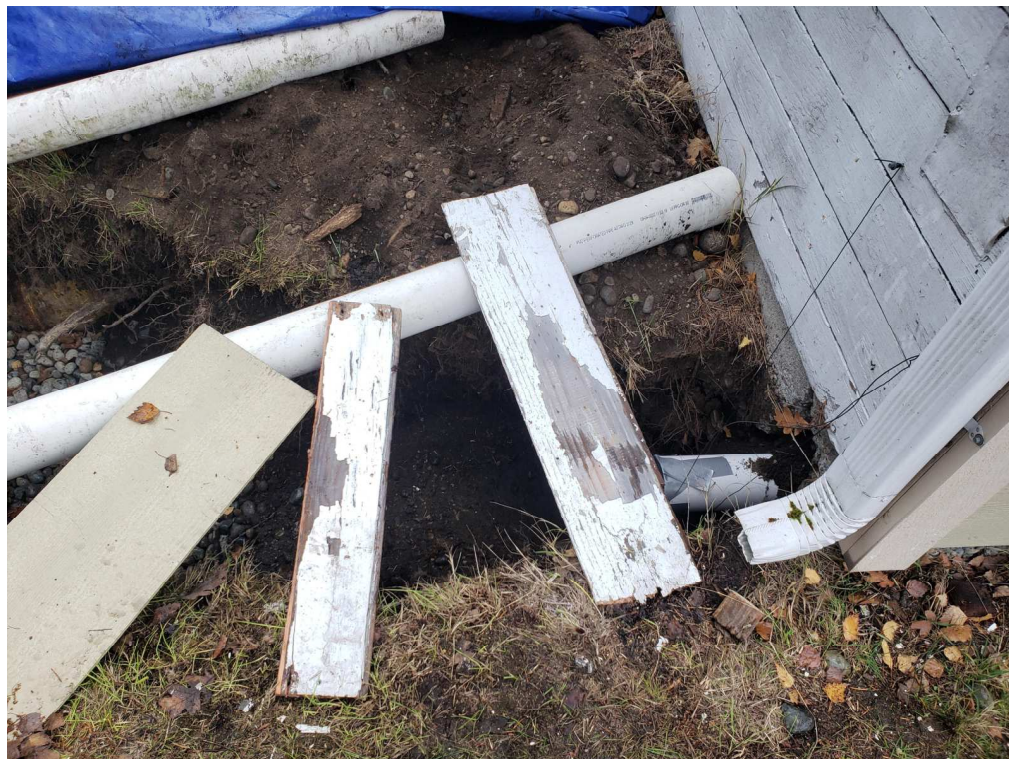
Fig. 2: 4 inch sewer pipe exiting the rear of the lab.
