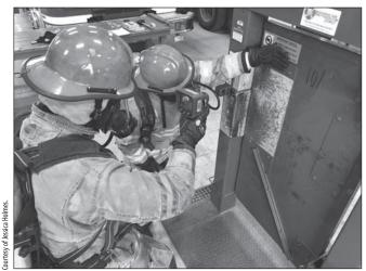
Look for any safety hazards as you evaluate the door. Inspect the door for the location and number of locks and their mechanisms.
