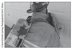
**3.** Starting at a center high point in the door, make a diagonal cut to the right, down to the bottom of the door.
