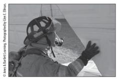
**5.** If necessary, pad or protect the cut edges of the triangle and the bottom panel to prevent injuries as fire fighters enter or leave the premises. If you have time, you can remove the cut portion of the door and the bottom rail by raising the bottom rail with a prying tool and then cutting the bottom rail in two places. (page 348)
