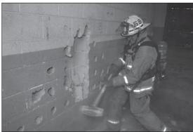
**3.** Knock out the remaining portion of the masonry blocks by hitting the masonry blocks parallel to the wall rather than perpendicular to it.
