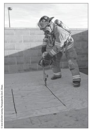
**2.** Use an appropriate cutting tool to cut one side of the hole. Cut the opposite side. Make two additional cuts at right angles to the first cuts. This will form a rectangle. Avoid cutting into the floor joists.
