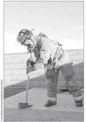
**1.** Size up the floor area, checking for hazards in the area to be cut. Sound the floor with an axe or similar tool to locate the floor joists.
