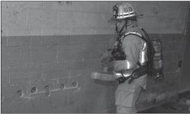
**1.** Size up the wall, checking for any safety hazards such as electrical outlets, wall switches, and plumbing. Inspect the overall area to ensure that the wall is not load bearing. Select a row of five masonry blocks at 2 to 3 ft (61 to 91 cm) above the floor. Using a sledgehammer, knock two holes in each masonry block. Each hole should pierce into the hollow core of the masonry blocks.
