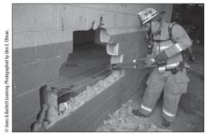
**4.** Clear any reinforcing wire using bolt cutters, and enlarge the hole as needed. (page 366)
